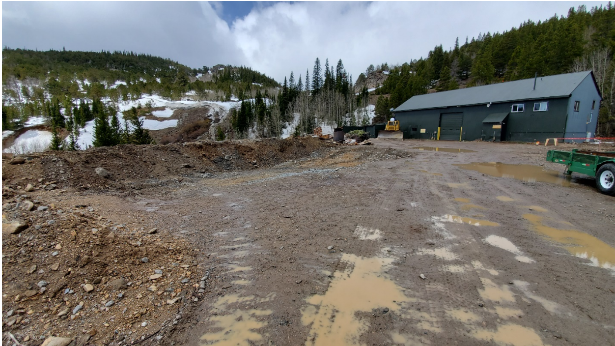
Caribou where old diesel containers were crushed has been cleaned/mitigated.
