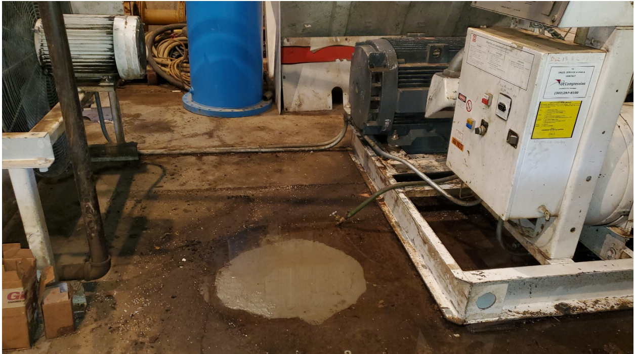
Ore building floor drain has been permanently sealed.
