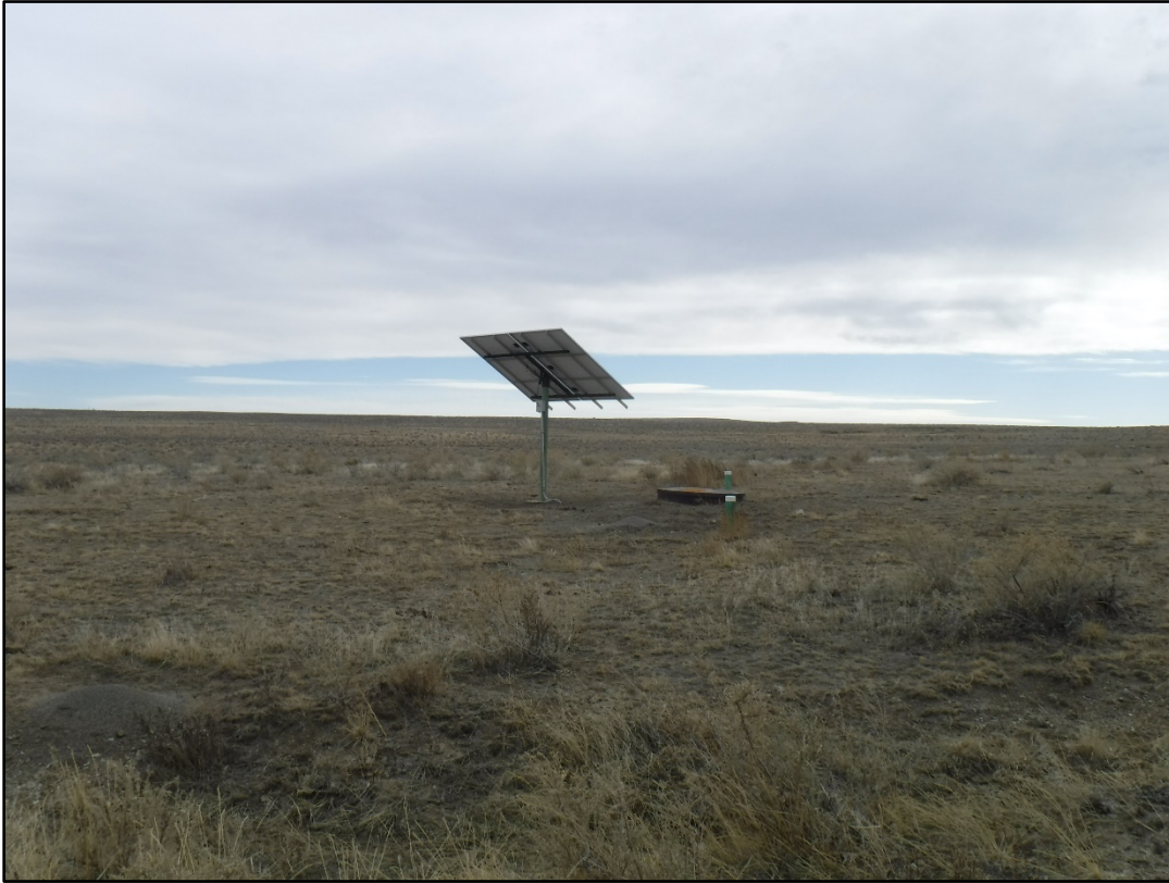
Photo 3: Solar powered booster station for cattle tanks
