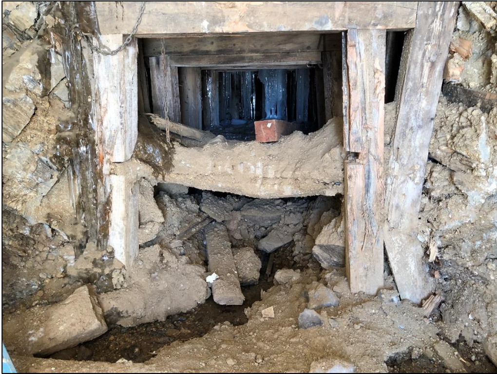
Photo 17. Closer view inside Caribou Mine portal, showing historic rotting timbers and large ice sheet hanging from roof inside adit.
