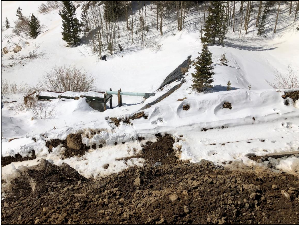
Photo 13. View looking west across area where three plastic lined ponds are present near Caribou Mine. A pipeline emerges from lower embankment of middle pond to discharge into lower larger pond. According to operator, these ponds have not been used in many years.
