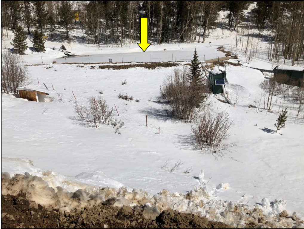
Photo 33. View looking northeast at lined pond #2 (indicated) where mine drainage from Cross Mine and Caribou Mine is directed before discharging at permitted outfall on Coon Track Creek. Note shed structures installed (at right) for water management system.
