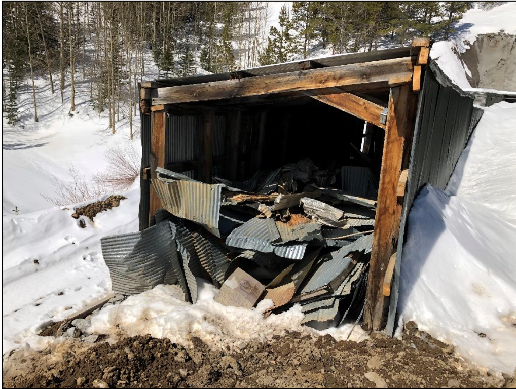
Photo 11. View of remaining portion of snowshed at Idaho Tunnel with scrap from demolished portion stored inside.
