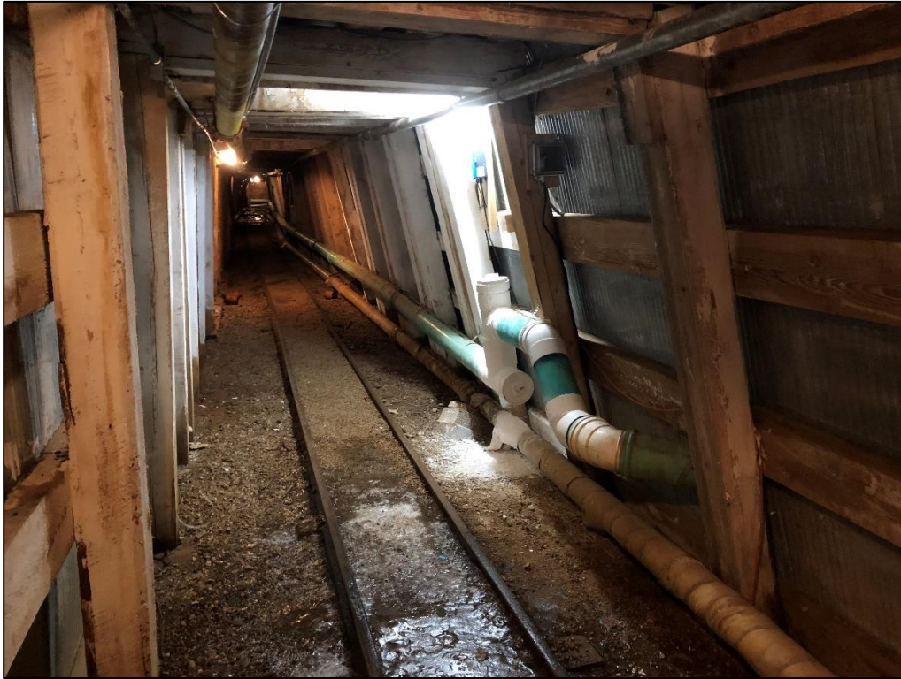
Photo 29. View looking northwest inside Cross Mine snowshed, showing pipe (at right) directing mine drainage to pond #1 for lime treatment. Note lit area (at right) where continuous flow meter is installed.
