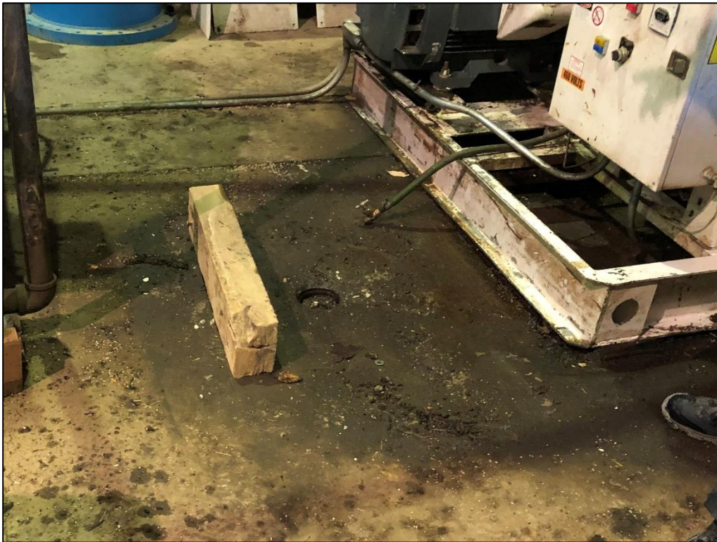
Photo 28. Closer view of floor drain inside Cross Mine warehouse building which must be permanently sealed if operator cannot describe how substances captured by this drain system are managed.
