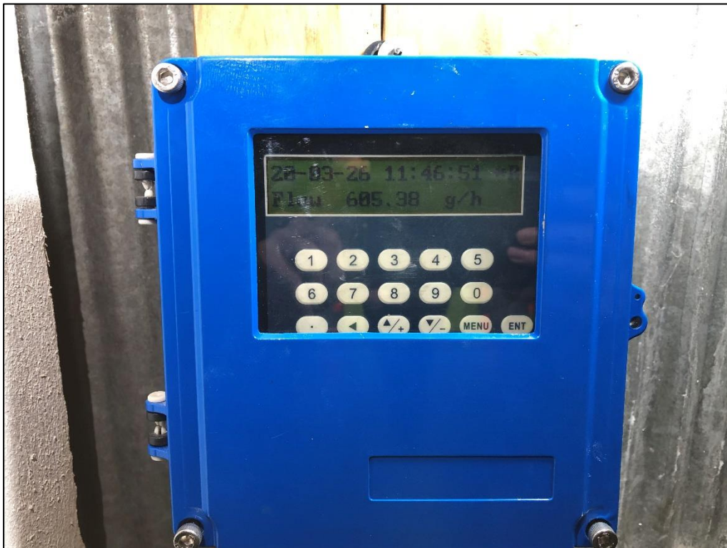
Photo 30. View of continuous flow meter installed inside Cross Mine snowshed to monitor discharge rate from this mine. Note discharge rate was 600 gph (10 gpm) during inspection. Caribou Mine discharge is measured by subtracting Cross Mine discharge rate from combined discharge rate at pond #2.
