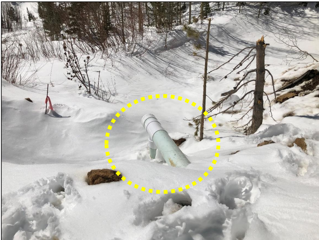
Photo 20. View looking southwest at new section of pipe (circled) installed to direct Caribou Mine drainage to pond #2, after old pipe was broken during excavation project.
