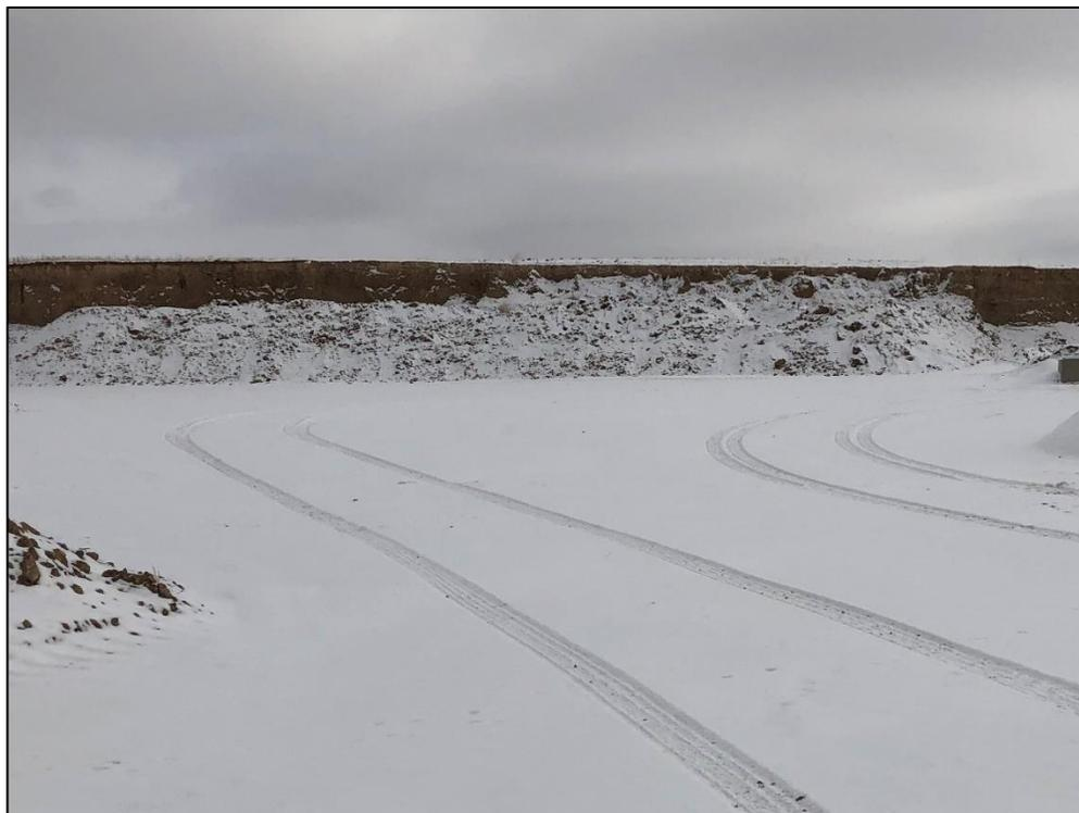
**Photo 18.** View looking east at eastern edge of mining Phases 3 and 4, showing pit walls approximately 12 feet in height with near vertical slopes.
