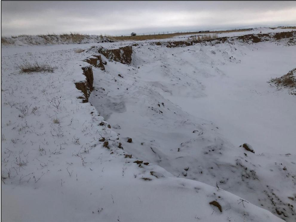
**Photo 7.** View looking southwest across most recently mined southeastern edge of pit (in mining Phase 3). Note highwall is approximately 12 feet in height with near vertical slopes.
