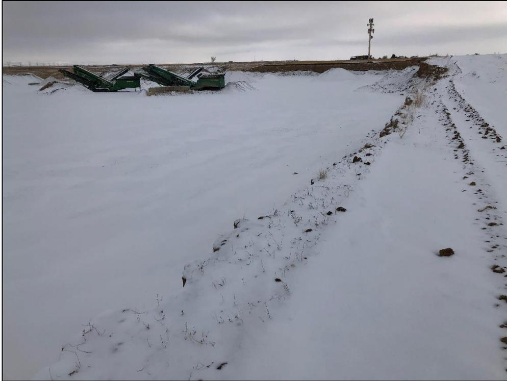
**Photo 9.** View looking north along eastern pit wall in mining Phases 3 and 4. Note pit wall approximately 12 feet in height with near vertical slopes.
