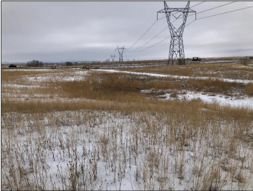
**Photo 1.** View looking west across Phase 2 mining area, showing slopes graded to 3H:1V or flatter and some grasses and annual weeds present in this area. Note transmission tower (at background right) located at western edge of permit area.
