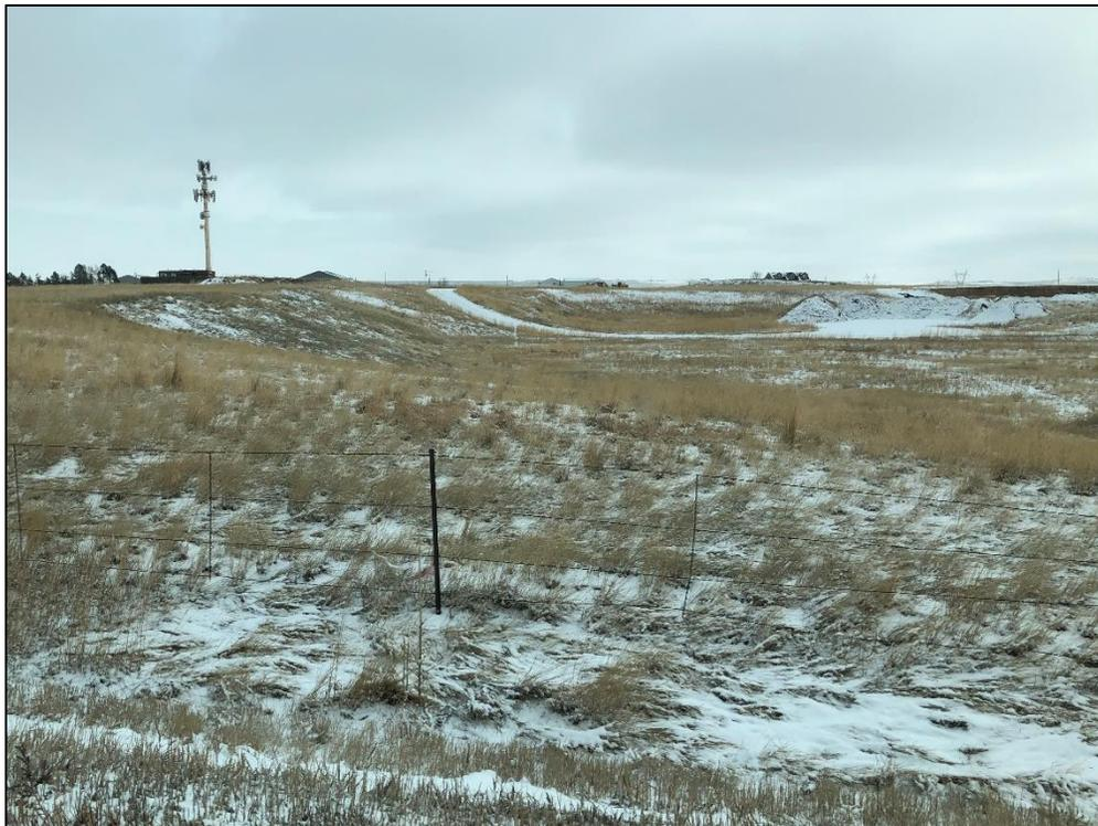
**Photo 20.** View looking east from western property line across northern edge of reclaimed mining Phase 1. Note slopes graded 3H:1V or flatter.
