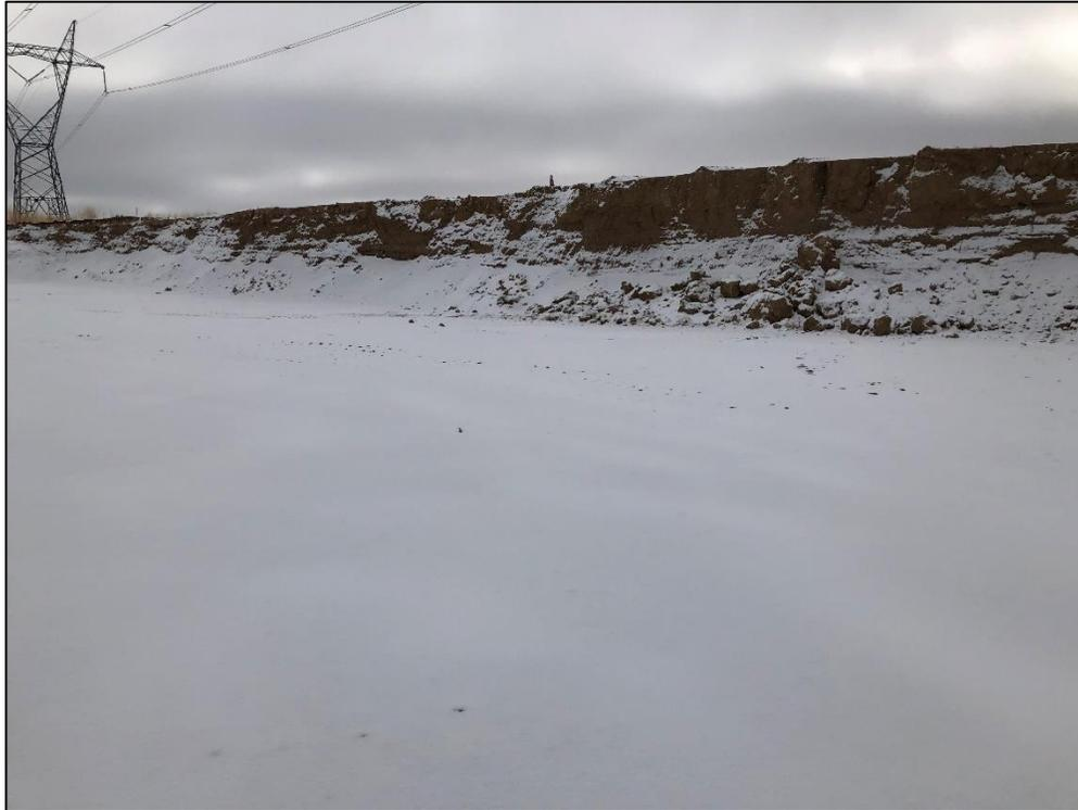
**Photo 17.** View looking southeast at southern edge of mining Phase 3, showing pit walls approximately 12 feet in height with near vertical slopes.
