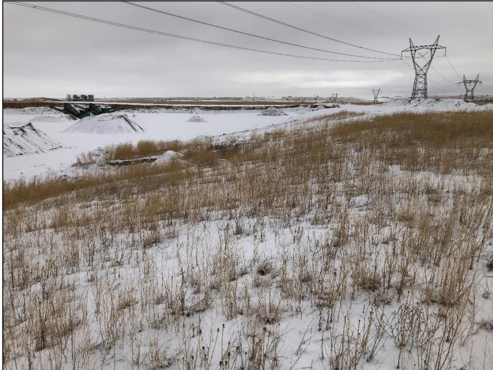
**Photo 3.** View looking east across southwestern pit wall in Phase 2 mining area, which has been graded to 3H1V.
