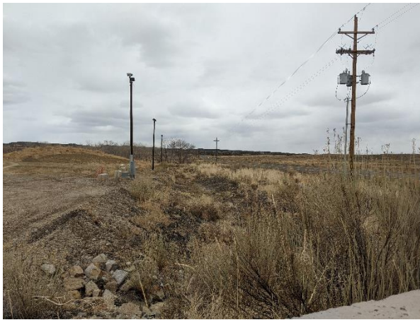
Photo 1: Ditch 1 looking east
