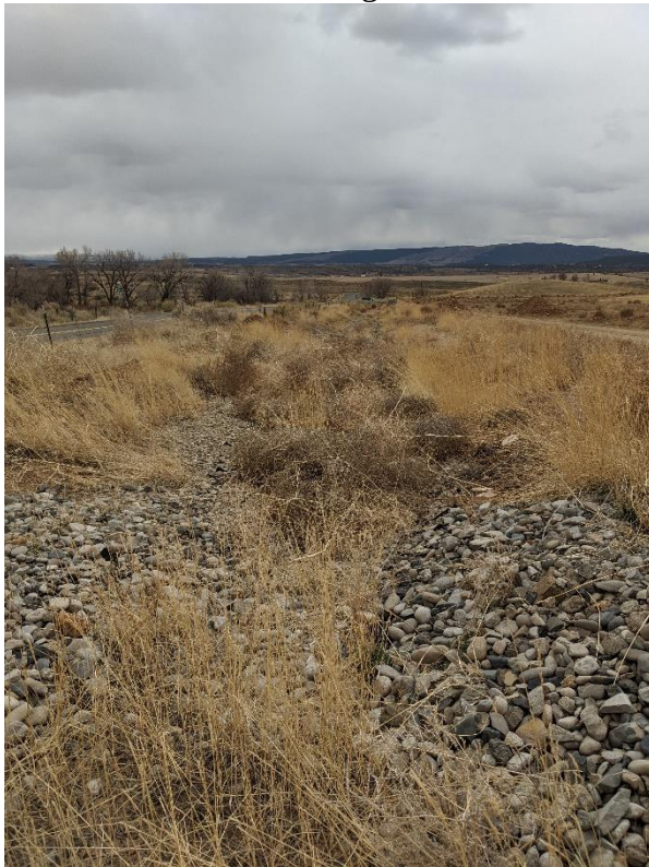
Photo 7: East ditch on east side of mine, looking south
