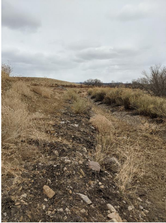
Photo 5: east ditch looking east
