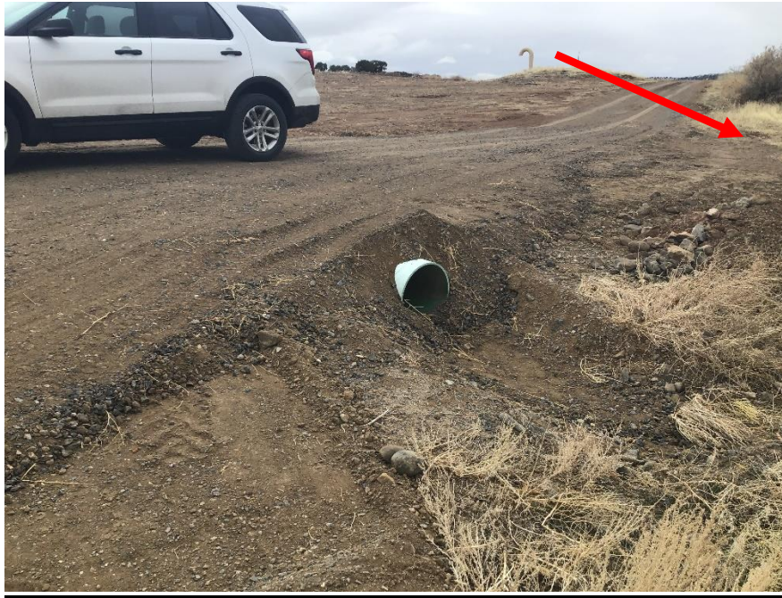
Photo 3: The photo above was taken as a follow up to previous Division inspections. The culvert shown above replaced a ditch noted in previous inspections located adjacent to the A Substation.
