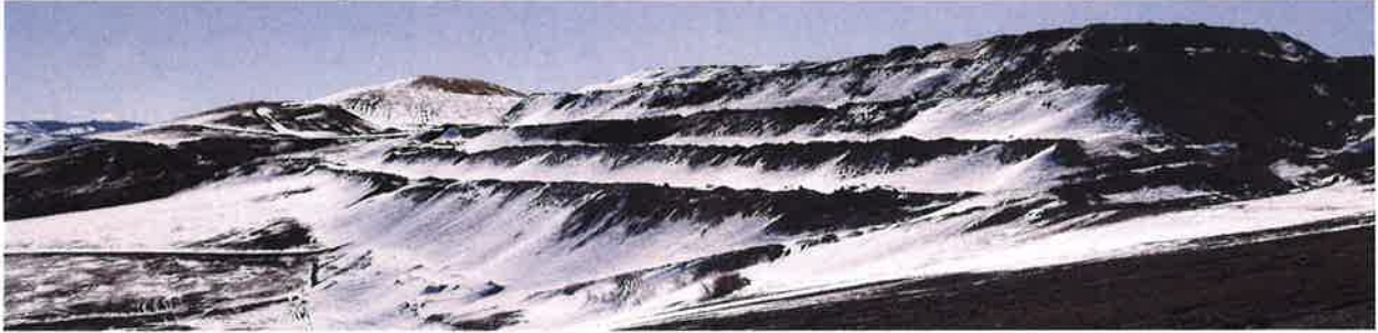
03-05-20 - East Taylor Fill looking east from the west ridgeline
