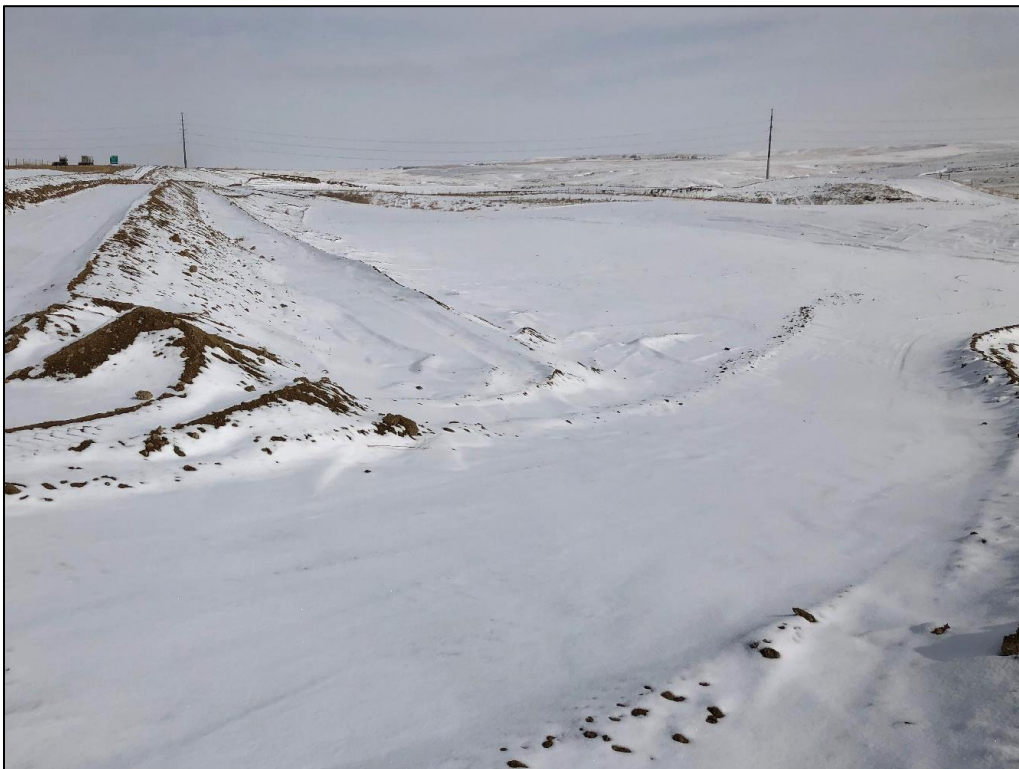
Photo 2. View looking north across western edge of southern mining area. Note pit wall slopes at approximately 3H:1V.
