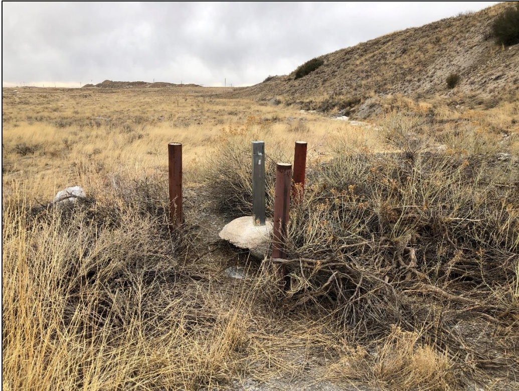
Photo 17. View looking south, showing monitoring well MW-1 located within A2-A CKD disposal area on top of small overburden mound. The well cap was secured with a padlock. However, the concrete apron around the well was elevated ~ 8 inches off the ground which could allow water to migrate down the casing and into the well. This needs to be repaired.
