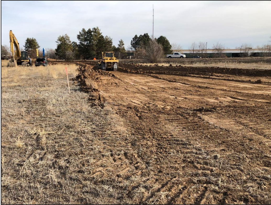
Photo 11. View looking southeast across northeastern corner of cell 21 which operation is stripping to create required visual berm along its eastern and southern edges prior to mining.
