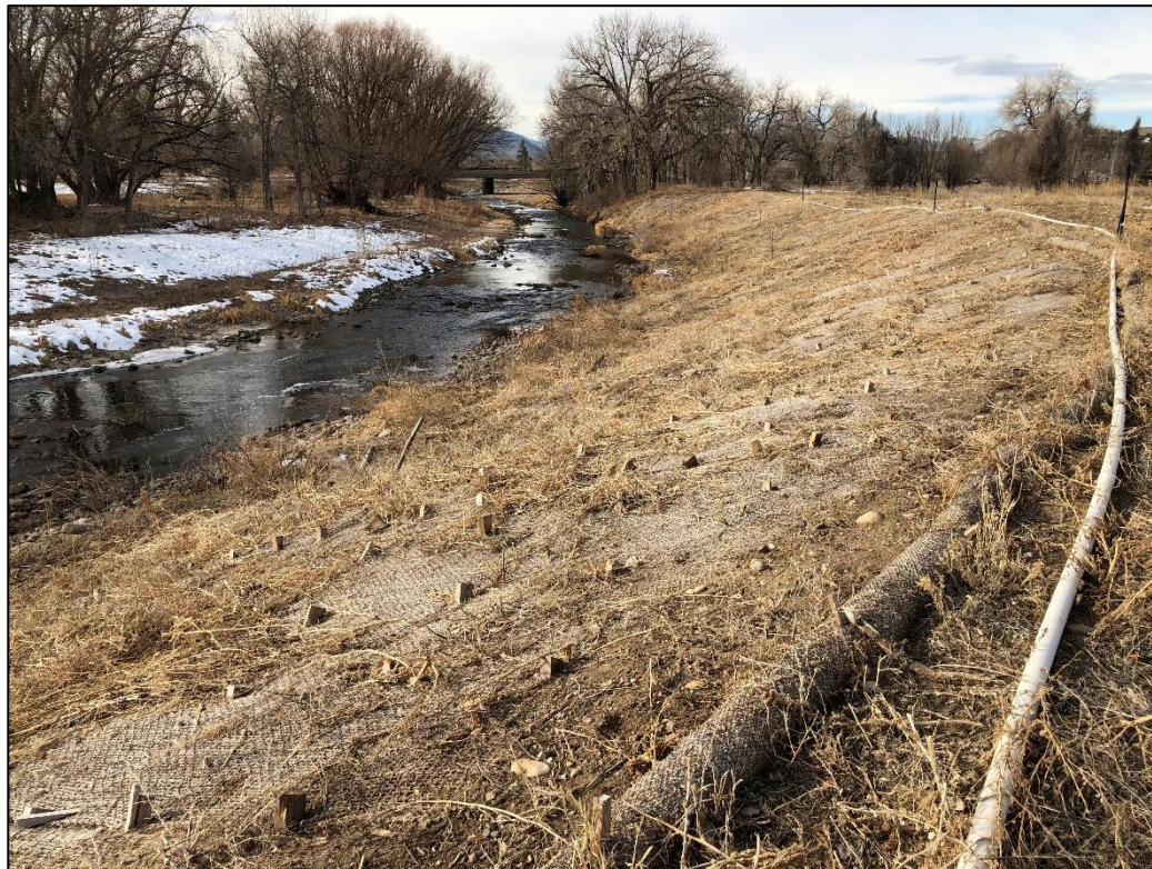
Photo 18. View looking northwest across northern river bank, showing erosion blanket, straw wattles, and irrigation pipeline (at right) installed by Big Thompson Watershed Coalition as part of river restoration project completed after September 2013 flooding.
