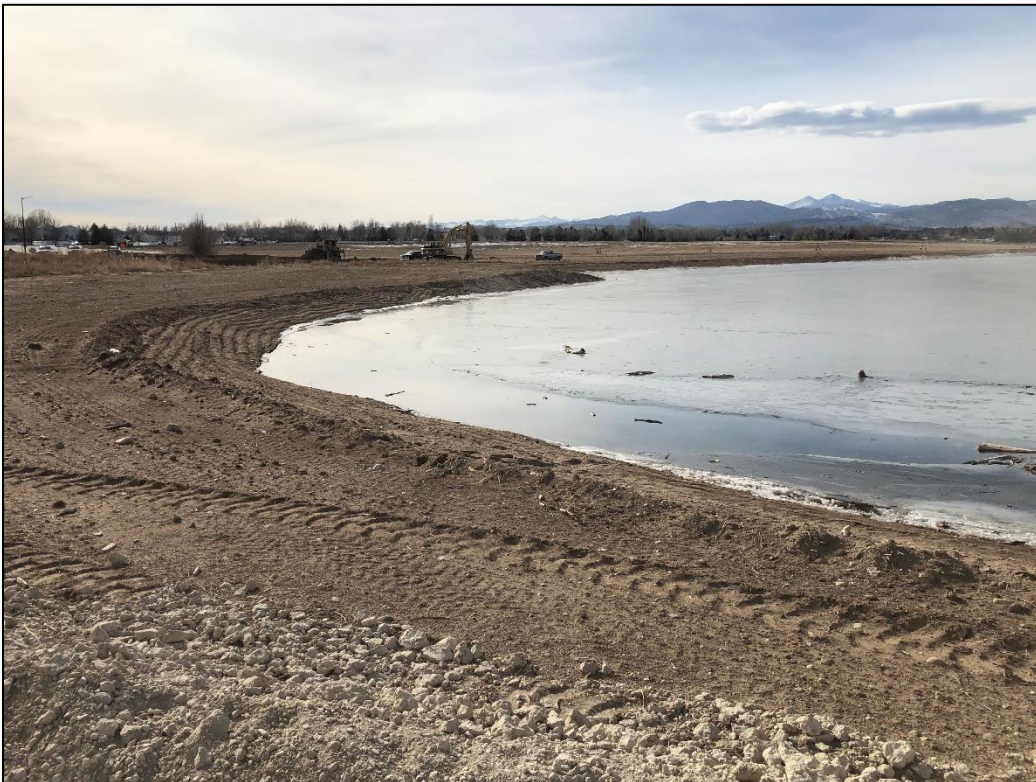
Photo 10. View looking southwest across eastern shoreline of cell 20, showing slopes graded 3H:1V or flatter.
