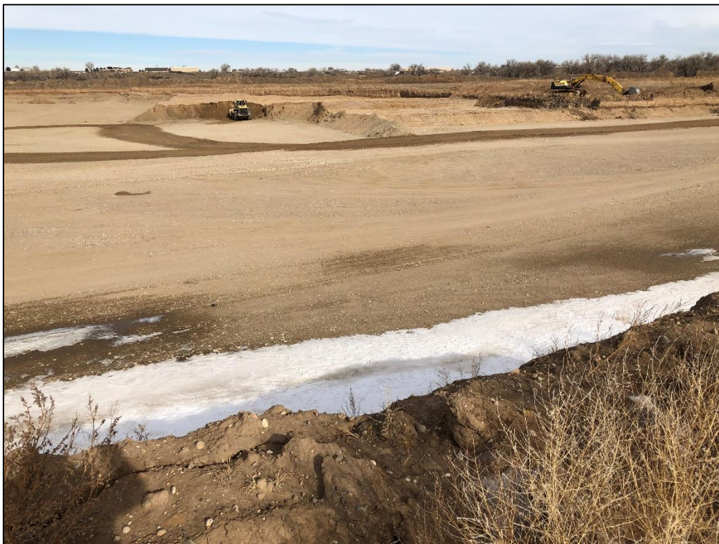
Photo 6. View looking northeast across Phase I Cell 2 pit, showing current excavation activities near center of pit, mining generally eastward.
