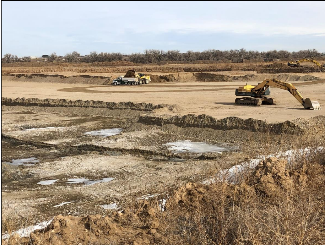
Photo 9. View looking northeast across Phase I Cell 2 pit, showing current excavation activities near center of pit, mining generally eastward.
