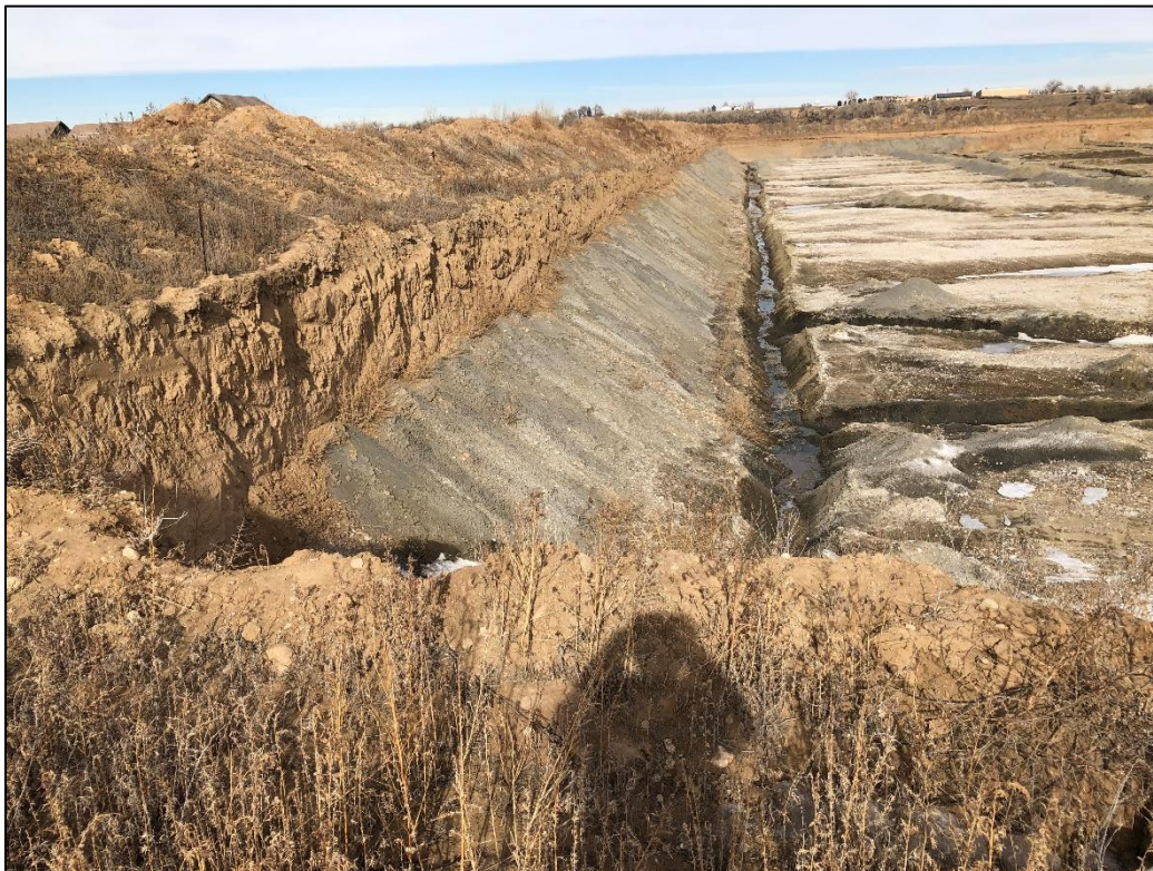
Photo 8. View looking north across western pit wall of Phase I Cell 2 pit, with slopes of 2.5H:1V (except for top 2-3 feet). Note topsoil bermed along top of pit wall.
