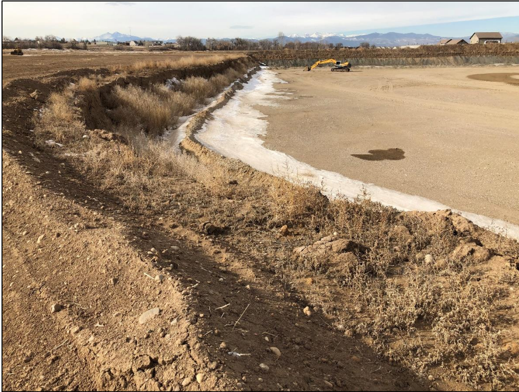
Photo 5. View looking west across south pit wall of Phase I Cell 2 pit, with slopes of 0.5H:1V to 1H:1V. This is considered an internal pit wall given its distance from the slurry wall, so its slopes can be steeper than 2H:1V.
