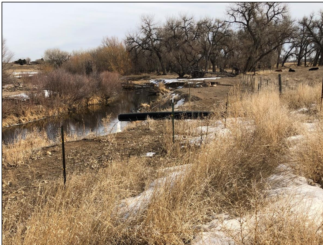
Photo 12. View looking east/southeast, showing sediment pond overflow pipe discharging water to river during inspection.
