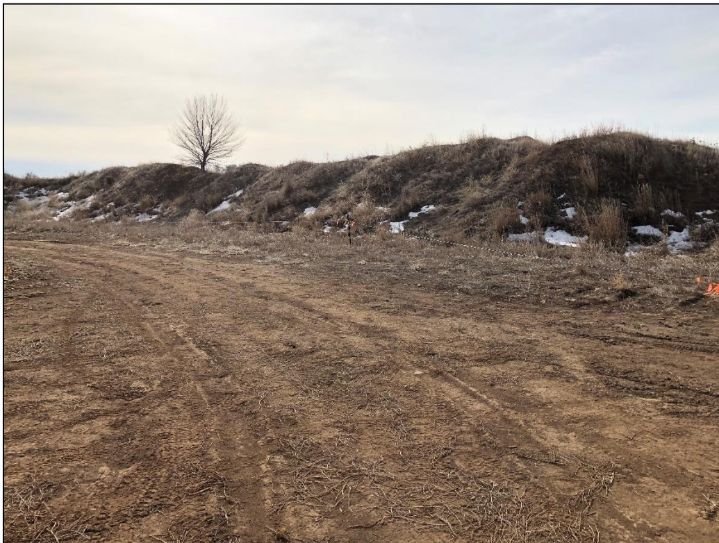
Photo 14. View looking south at topsoil bermed along northeastern edge of Phase I Cell 2 pit. This stockpile was stable with good grass cover.
