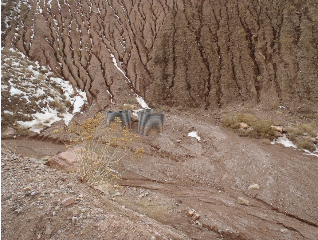
Photo 4. Rilling above sediment control Pond No. 2 (looking west).
