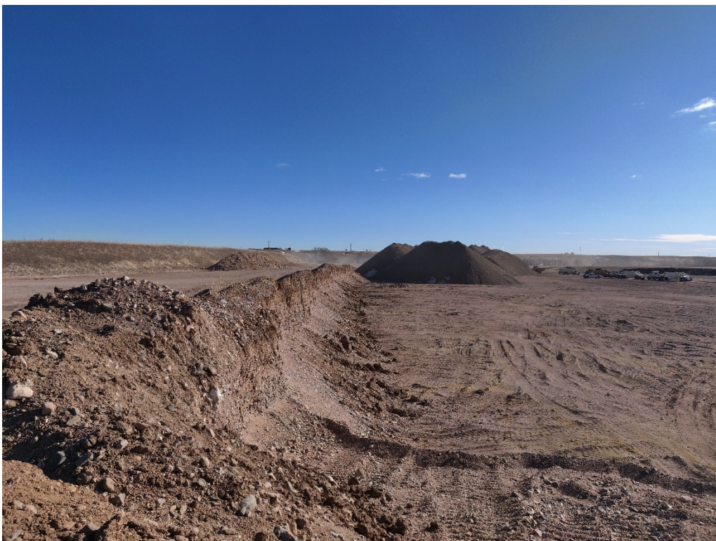
View of the north highwall and pit floor from the northwest highwall looking east
