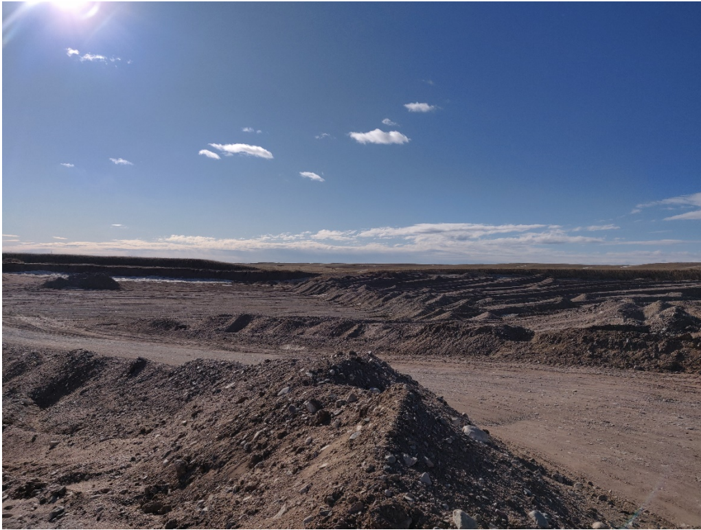
View of the current excavation area located in the southwest corner of the site
