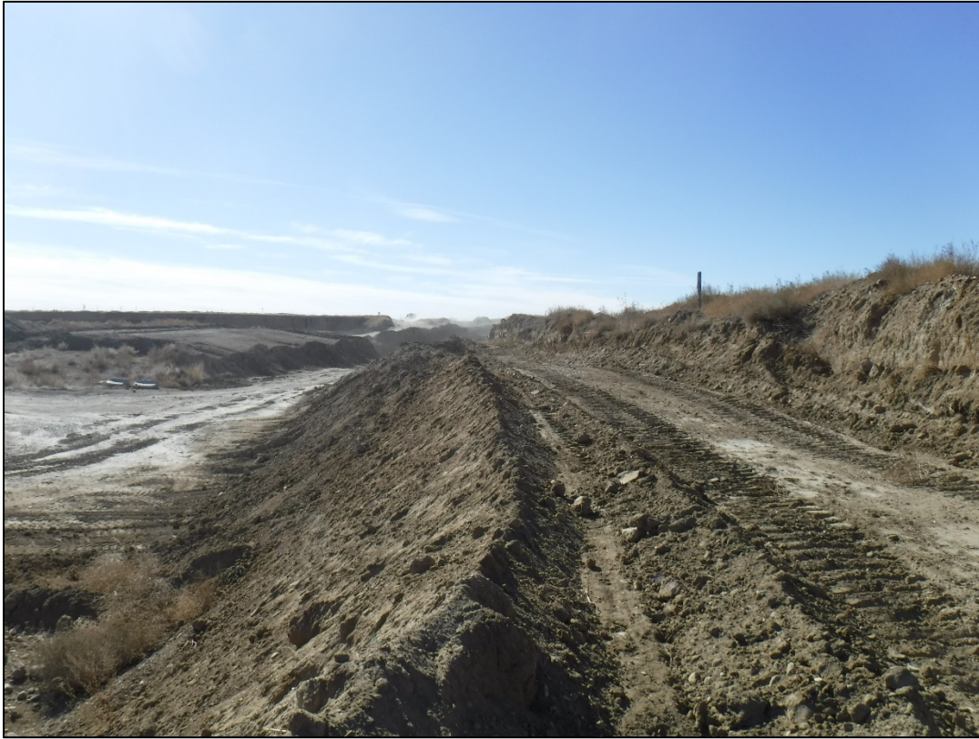
Photo 9: Reclaiming the slope adjacent to Cesar Road to a 3H:1V grade.
