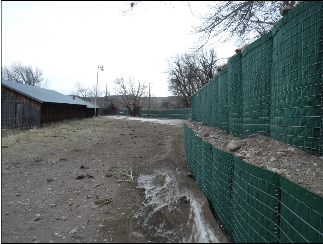
Photo 5: Looking east along the flood barrier wall after the stacking has begun
