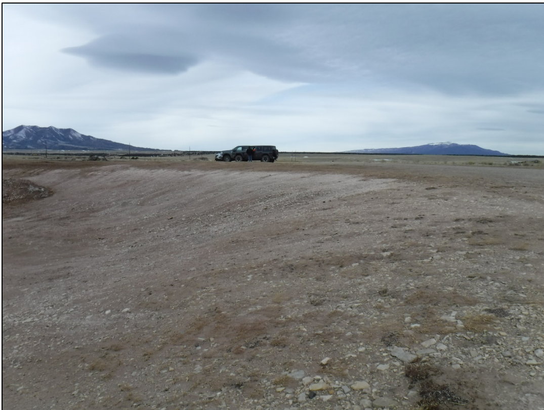
Photo 12: Eastern end of pit with side slopes graded to a 3H:1V slope
