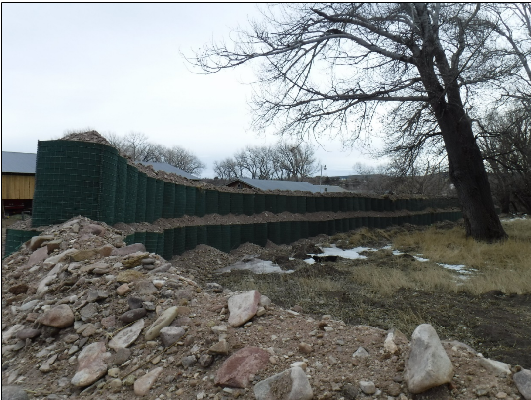
Photo 4: Looking east along the flood barrier wall about half way along the overall length where the flood barrier wall is stacked
