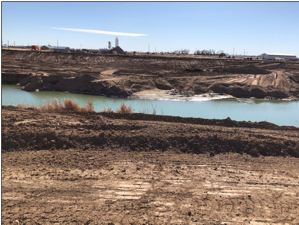
Photo 10. View looking south across central portion of Pond D from its northern edge, showing backfilled southern edge of pond to existing island (in background).
