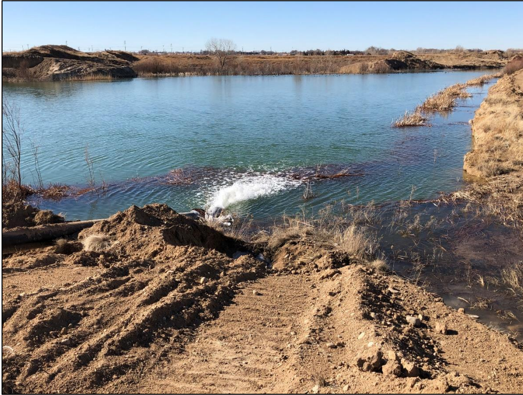
Photo 7. View looking southwest across Pond C from its northeastern corner, showing above-ground pipeline discharging water pumped from Pond D.
