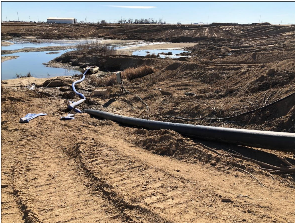
Photo 6. View looking southeast across Pond D, showing dewatering pump and above-ground pipeline located at its northwestern corner.
