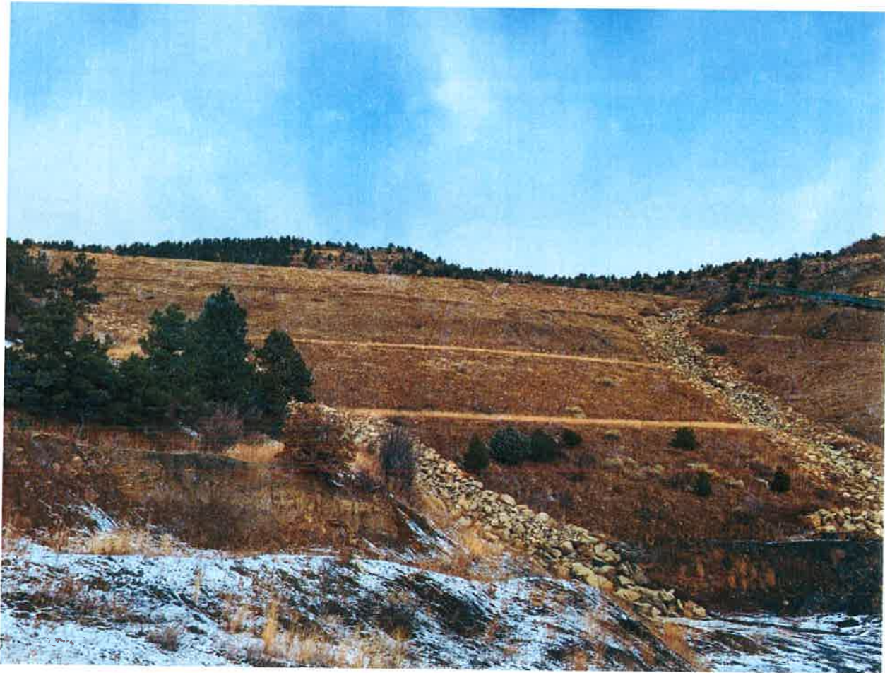
Refuse Disposal Area – Reclaimed Benches and Armored Drainage
