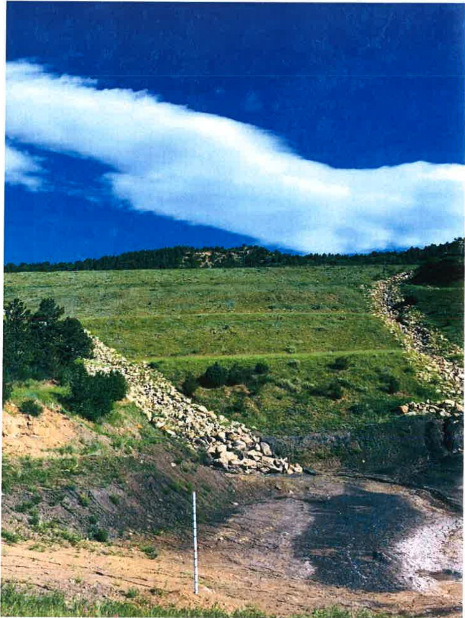
Refuse Disposal Area – Reclaimed Benches and Armored Drainage – September 19, 2019
