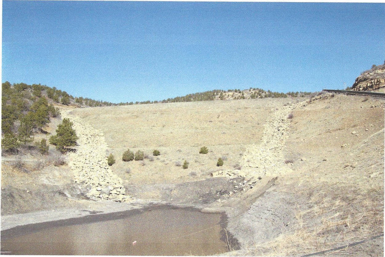
Refuse Disposal Area – Reclaimed Benches and Armored Drainage – March 29, 2019
