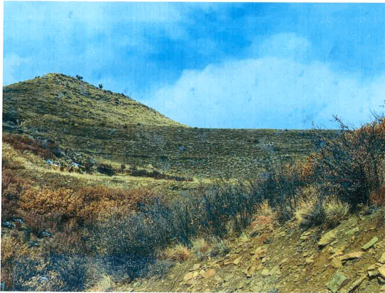
Fill 9 – South Facing Embankments
