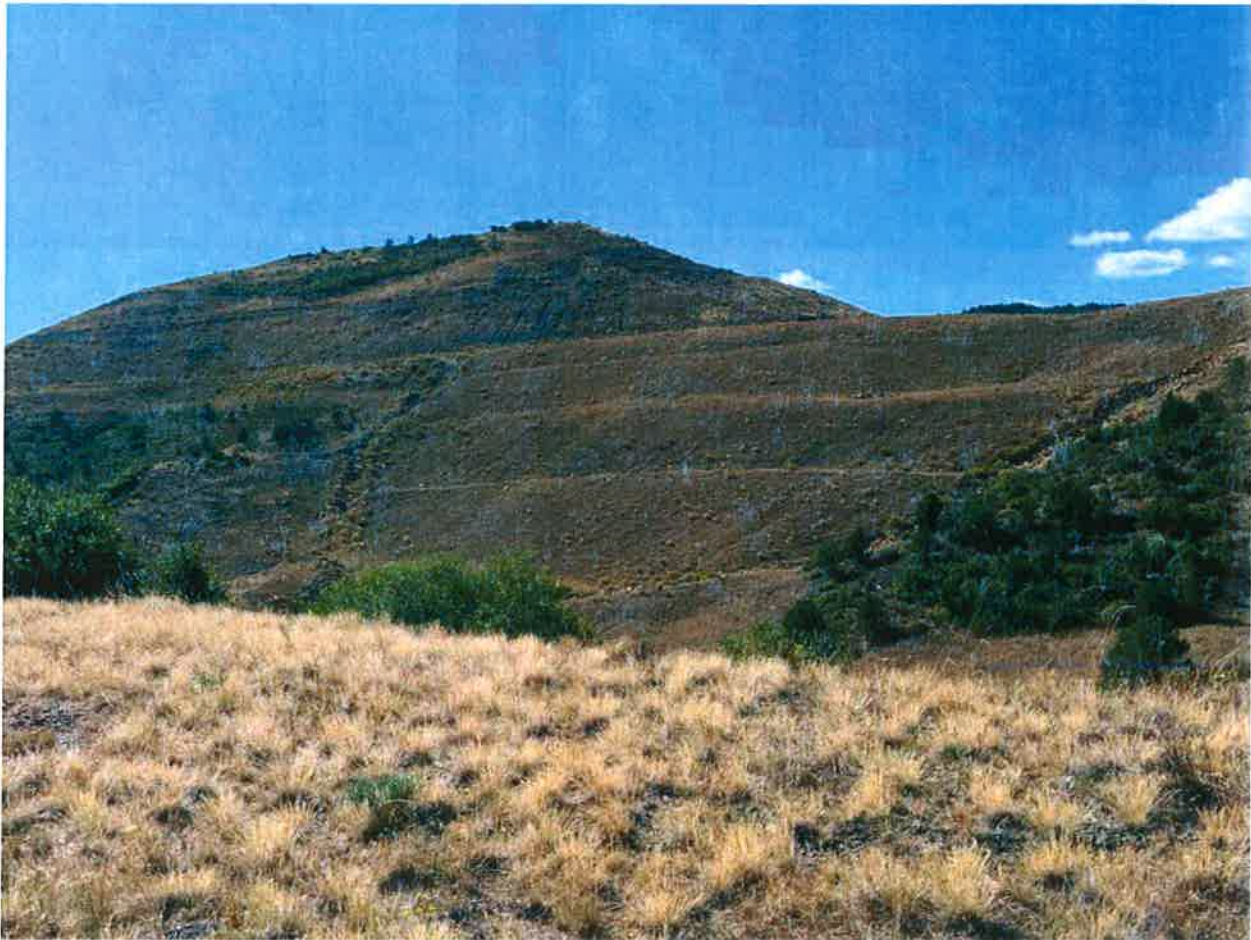
Fill 8 - North Facing Embankments with Down Drains Visible
