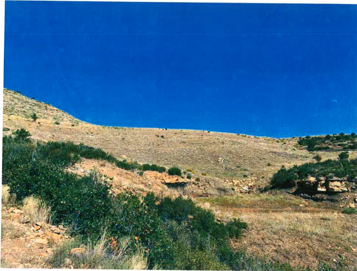
Fill 9 – South Facing Embankments
