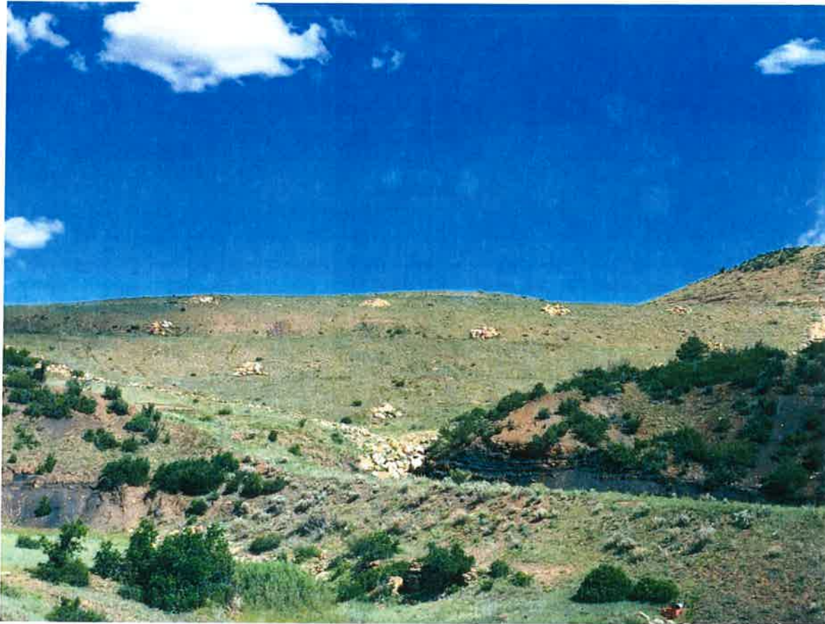
Fill #7- South Facing Embankments
