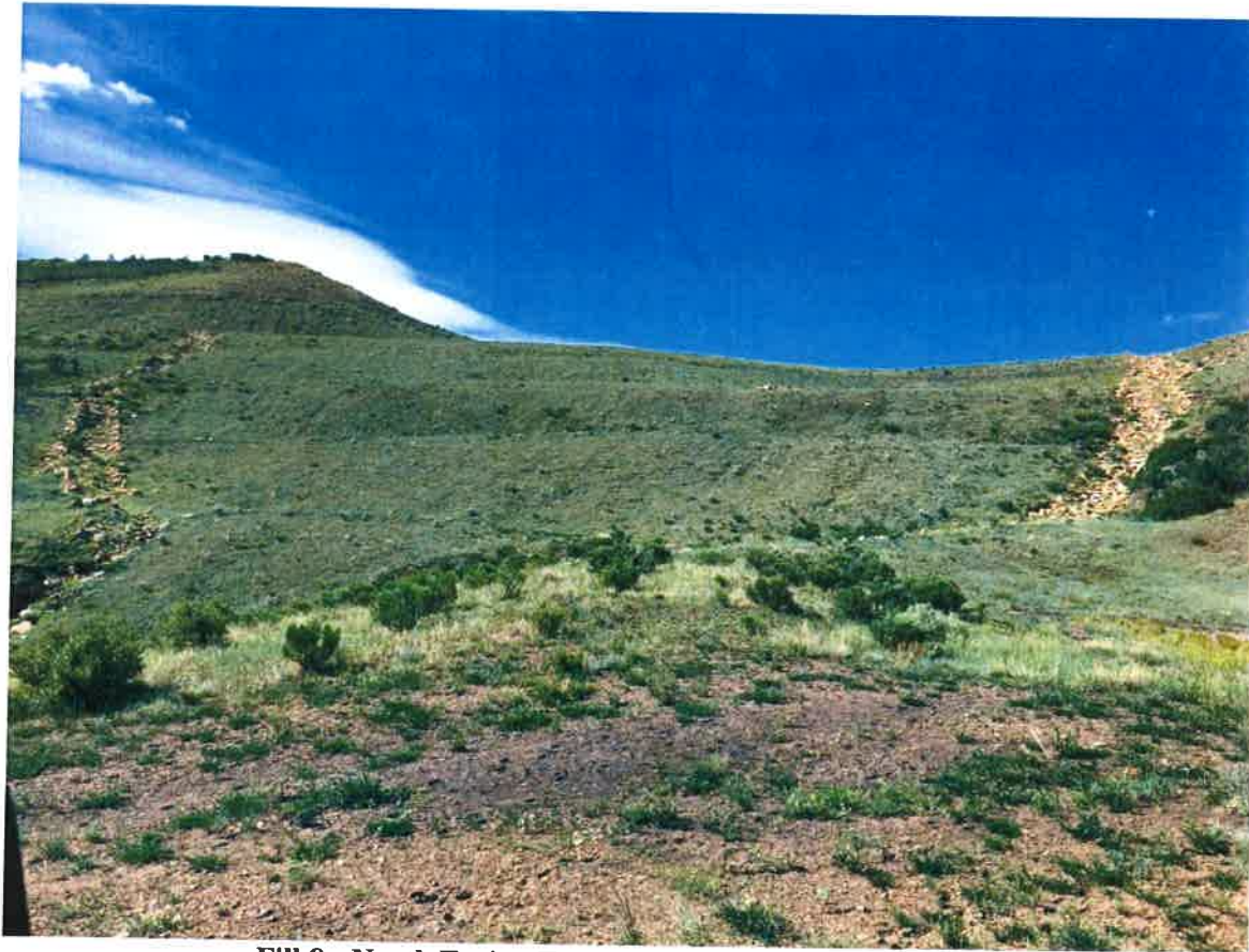
Fill 8 - North Facing Embankments with Down Drains Visible
