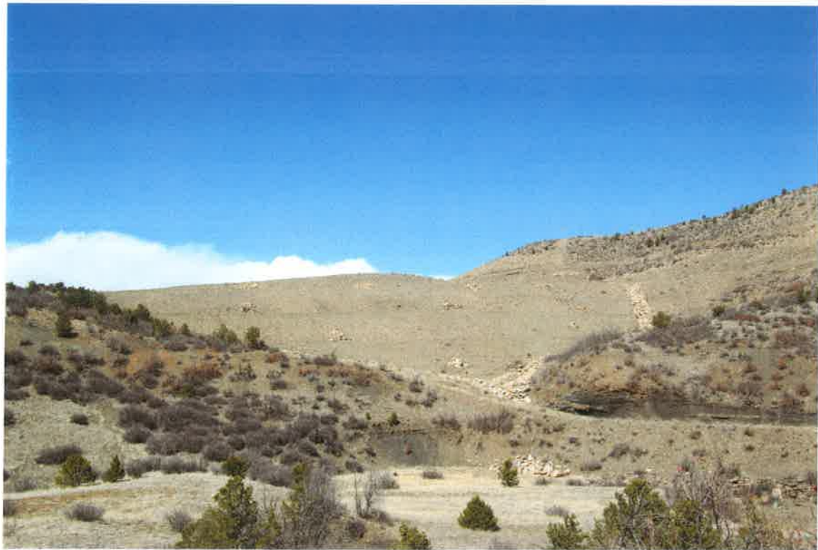
Fill #7 – South Facing Embankments with East Armored Down Drain Visible
