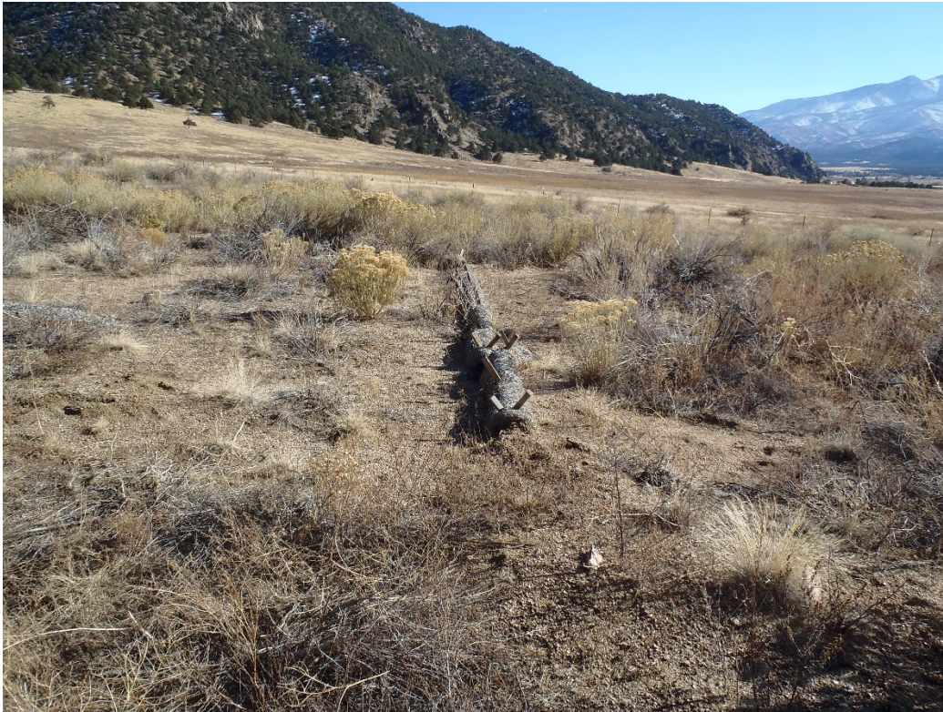
Photo 6. Straw wattles downgradient of pit near SW corner (looking SE).
