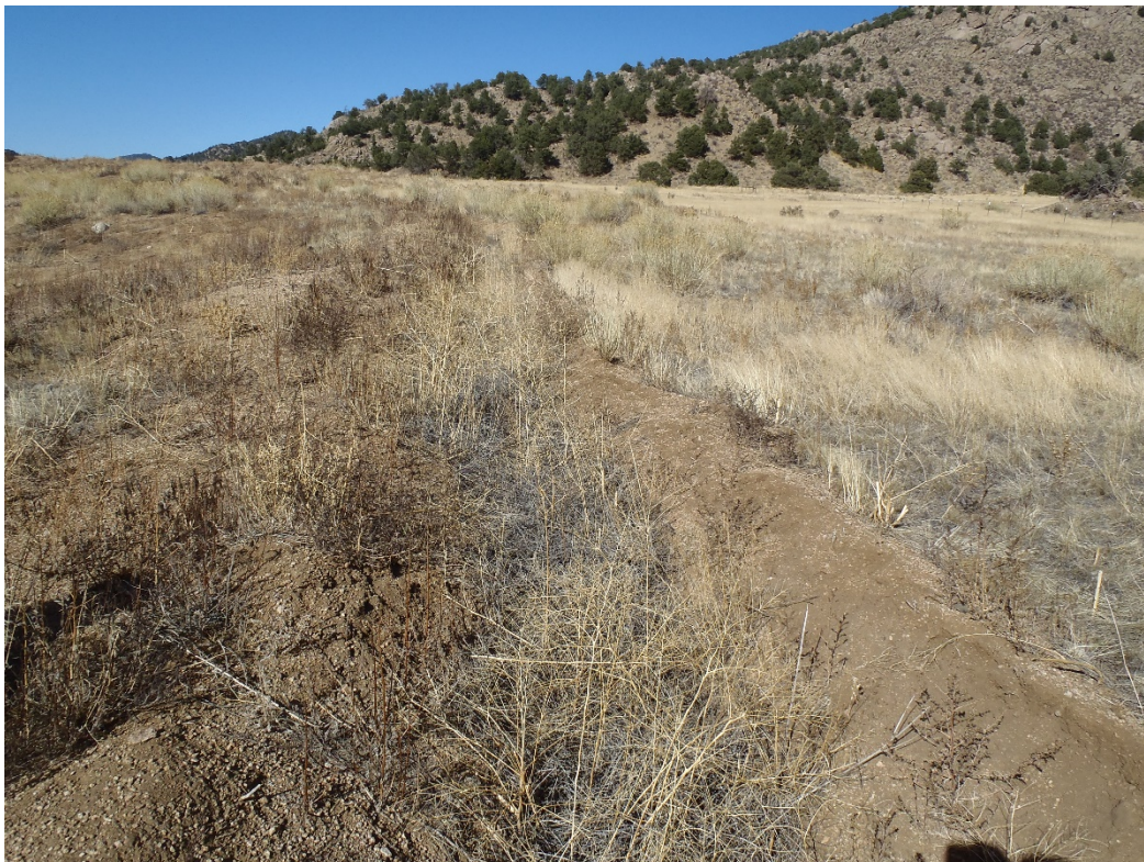
Photo 5. Diversion ditch on east side – needs some maintenance (looking north).
