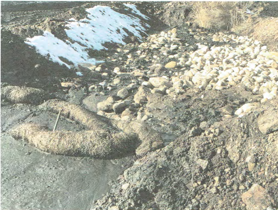
Pic. 4 – Erosion control above area inlet of Reach 7/under-drain interface.
