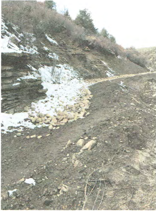
Pic. 3 – New clean water channel for Reach 3 relocation.
