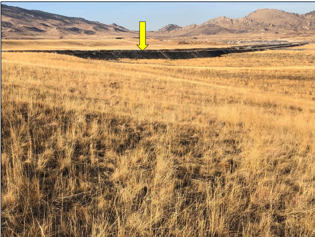
Photo 12. View looking northeast across reclaimed area located south of active mining area, with slopes graded 3H:1V or flatter and established grass cover. Note road constructed along northern edge of this area (indicated) to access 3 rd Ridge pit.
