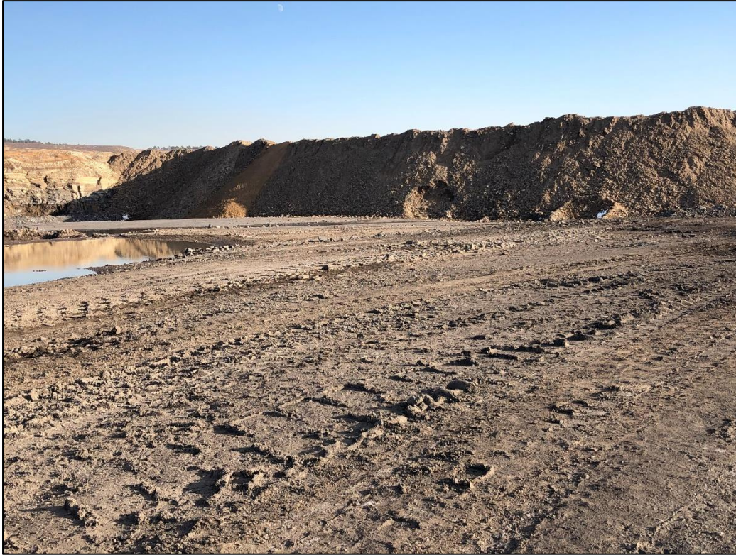
Photo 13. View looking south across 3 rd Ridge pit, showing backfilled southern portion of pit which will need to be retopsoiled and seeded once final grading is complete.
