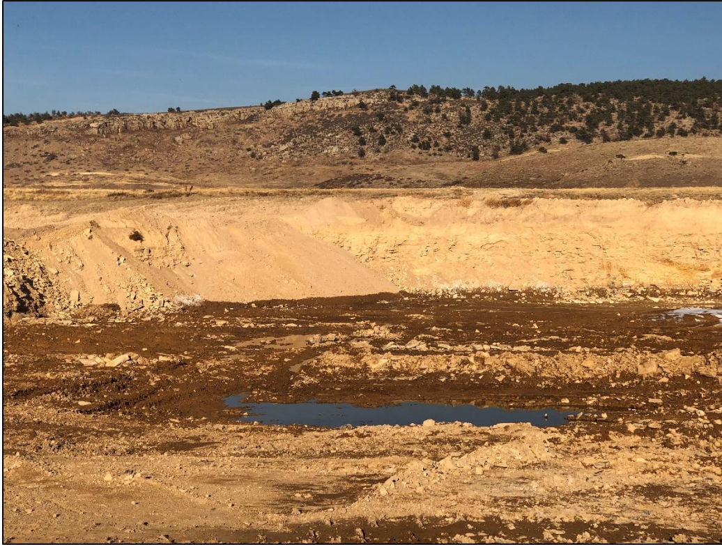
Photo 19. View looking north across 4 th Ridge pit, showing northern pit wall approximately 15 feet in height with near vertical to 1H:1V slopes.
