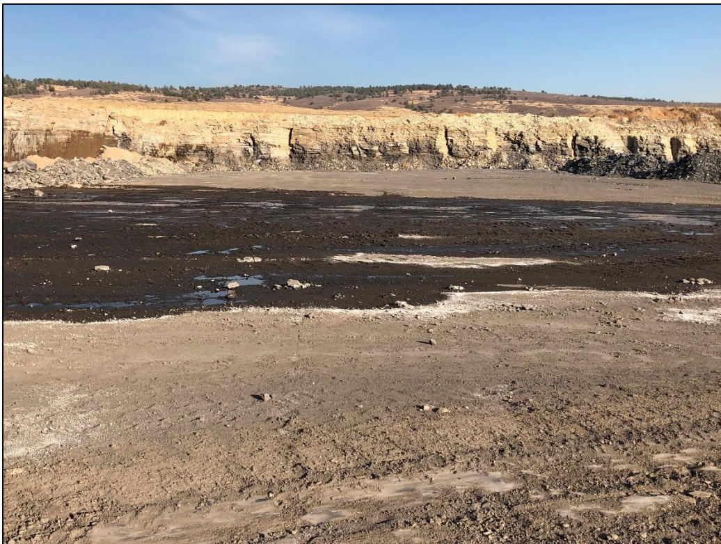
Photo 14. View looking east across 3 rd Ridge pit, showing eastern pit wall (in background), approximately 20-25 feet in height with near vertical slopes.
