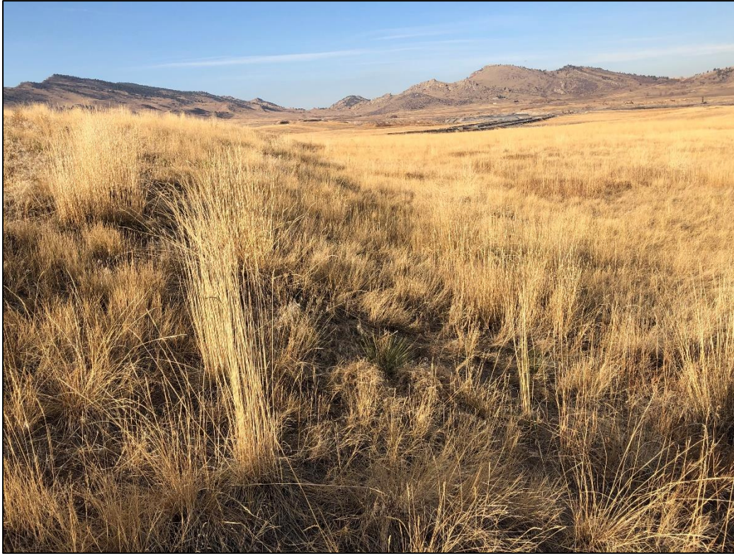
Photo 11. View looking north across reclaimed area located south of active mining area, with slopes graded 3H:1V or flatter and established grass cover.
