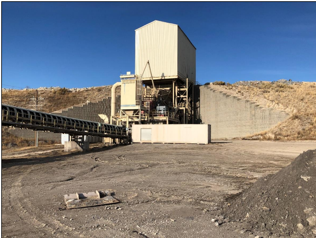
Photo 4. View looking north at crusher facility located near main haul road, south of active mining area. Note crusher is enclosed in a metal housing.
