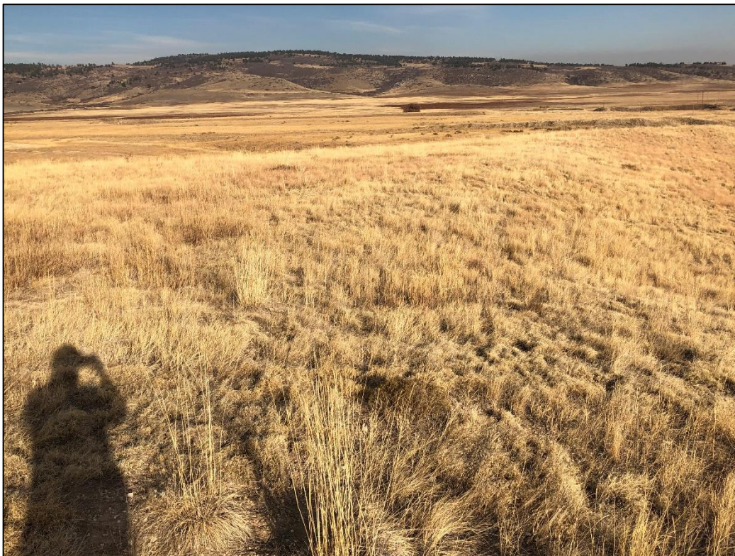
Photo 10. View looking east across reclaimed area located south of active mining area, with slopes graded 3H:1V or flatter and established grass cover.
