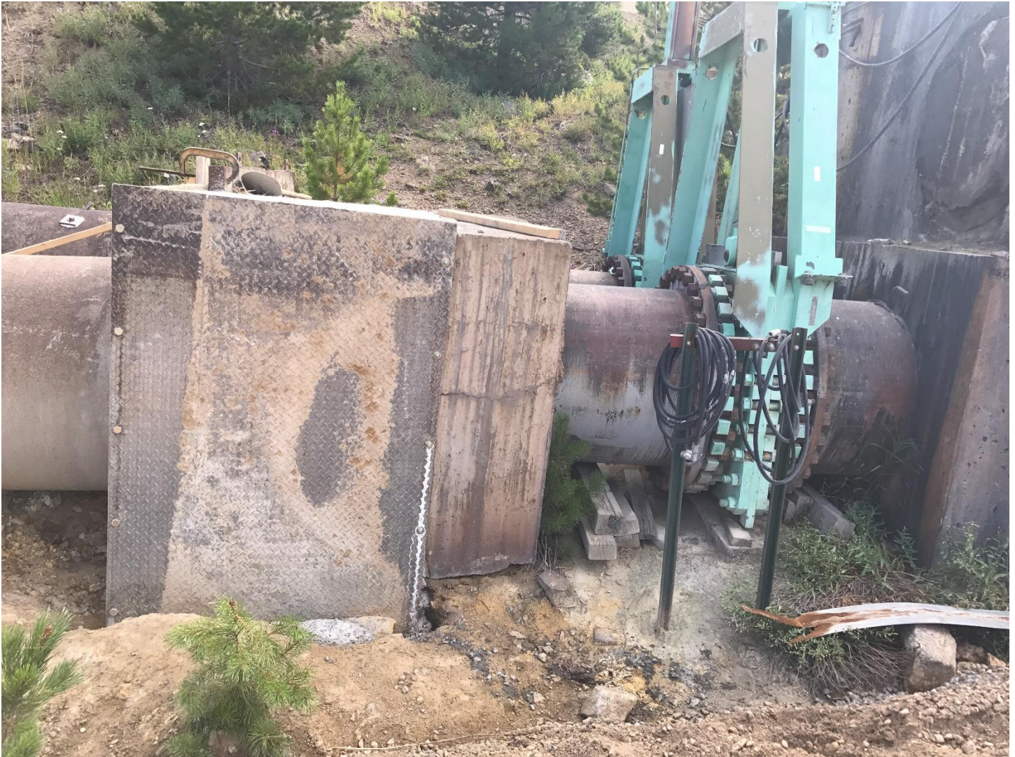
Concrete Form around pipe joint- source of leak
