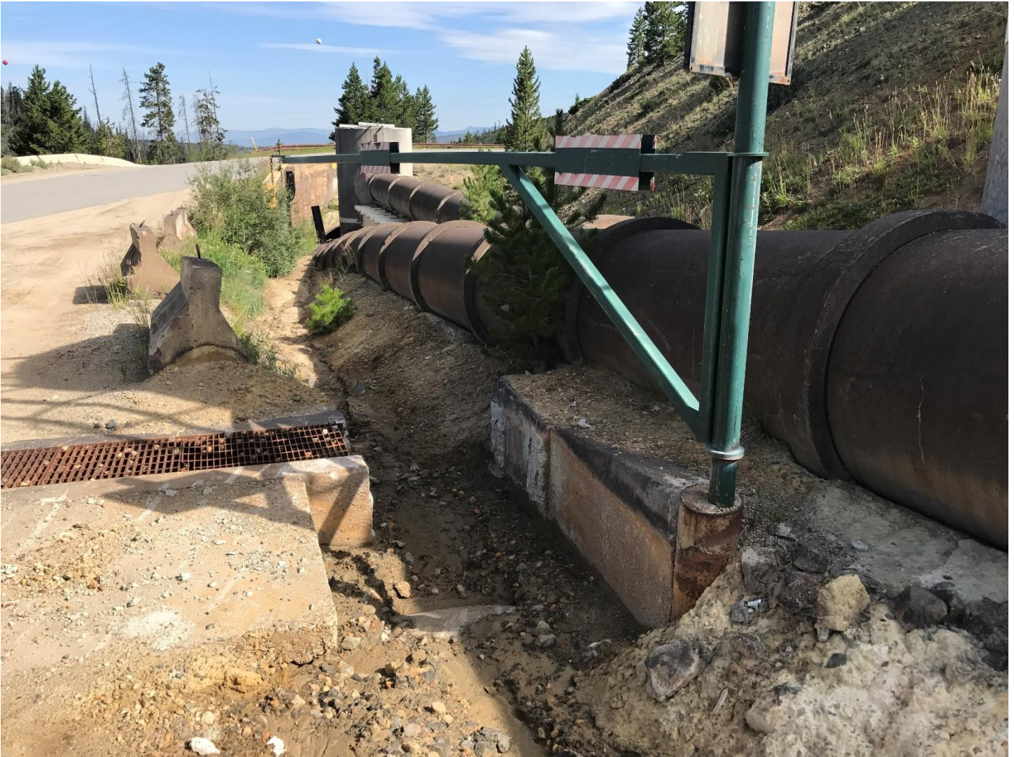
Leak area- ditch where water was conveyed
