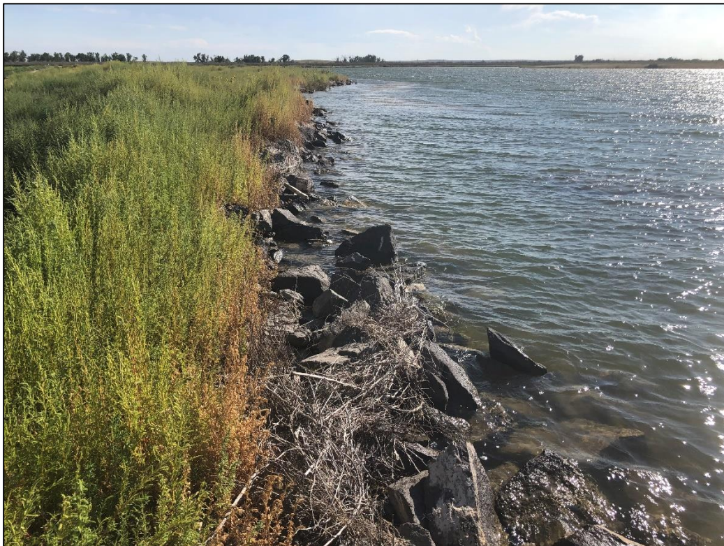
Photo 16. View looking south across eastern pond shoreline with riprap installed per TR-6. The riprap appears to be effectively controlling erosion along this portion of the shoreline.
