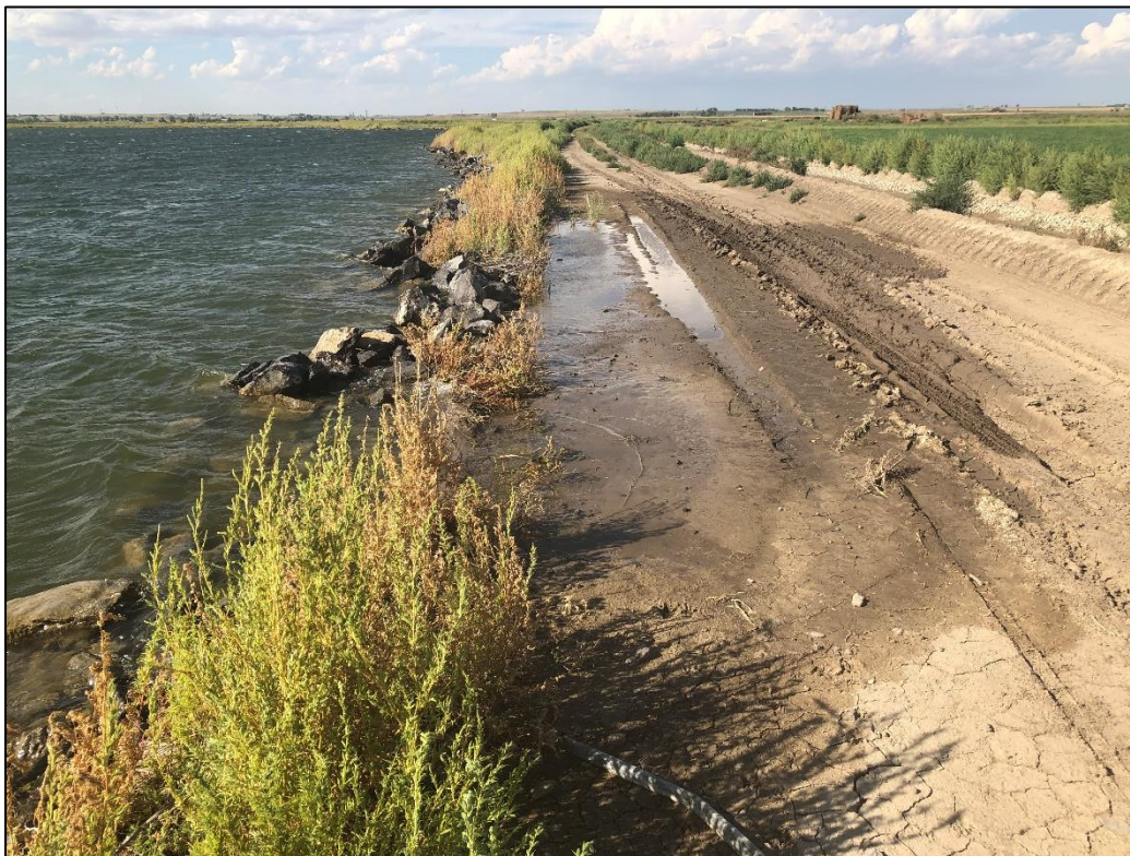
Photo 18. View looking north across portion of eastern pond shoreline where riprap placement is not effectively controlling erosion. Note pond water is overflowing bank onto adjacent farm road.
