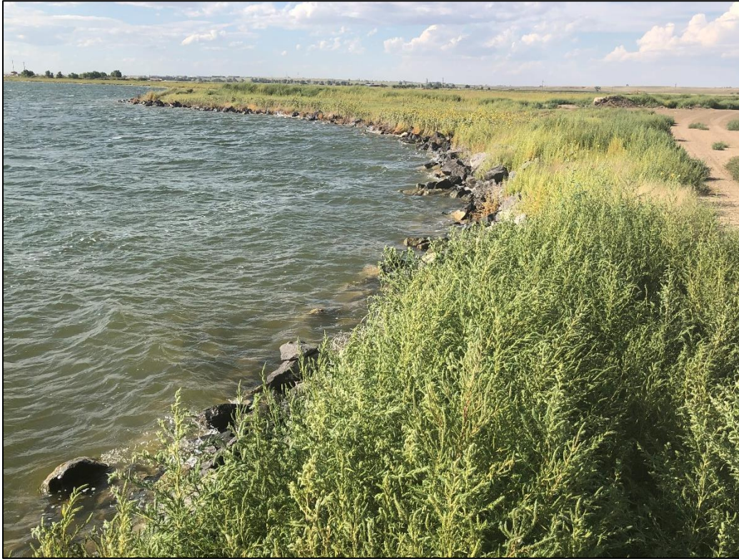
Photo 17. View looking north across eastern pond shoreline with riprap installed per TR-6. The riprap appears to be effectively controlling erosion along this portion of the shoreline.
