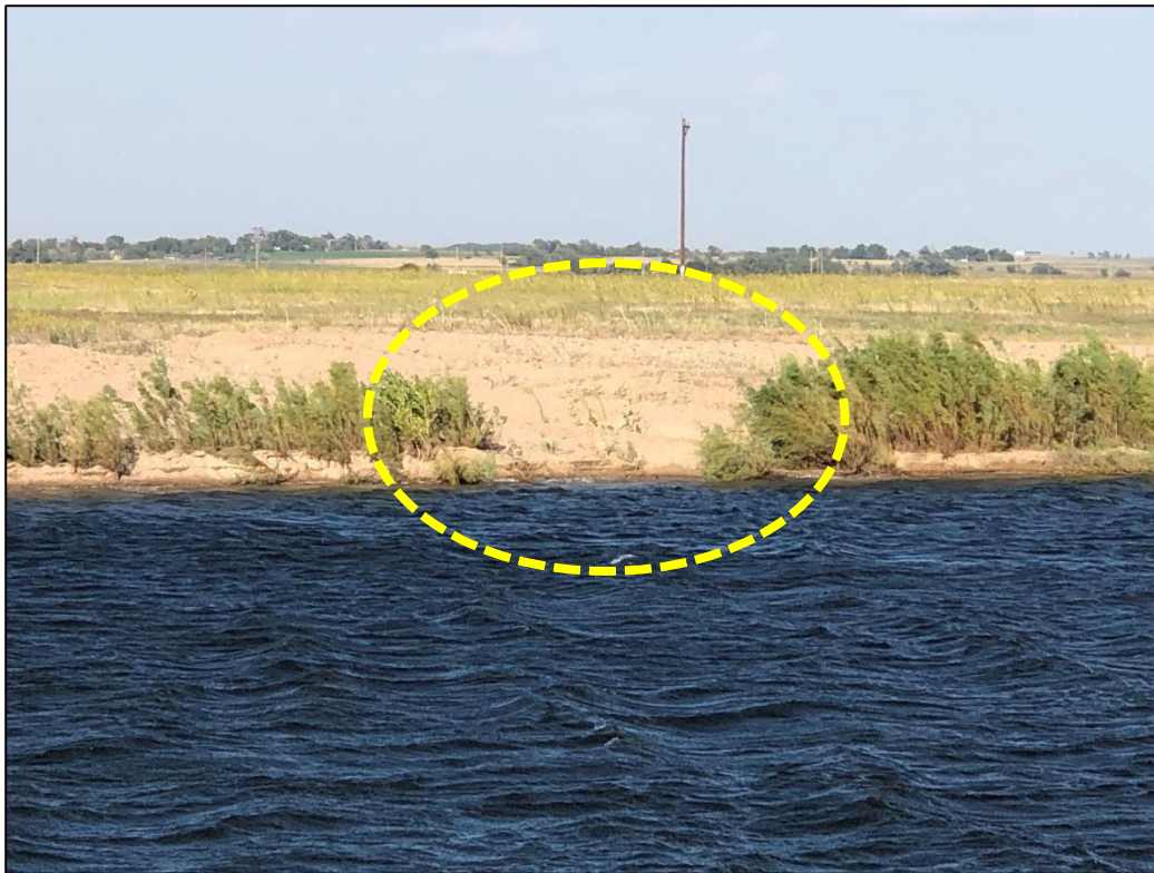
Photo 31. View looking east across northwestern portion of pond, showing erosion feature (circled) observed along northern pond shoreline.
