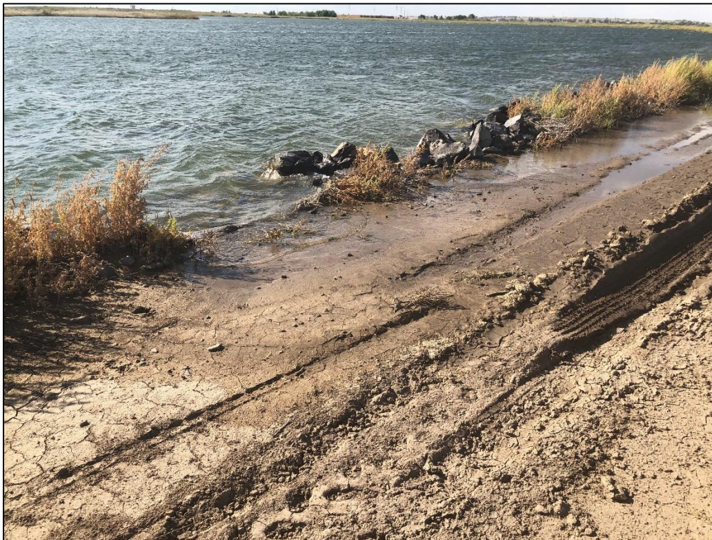
Photo 19. Closer view of area shown in Photo 18, looking northwest across portion of eastern pond shoreline where riprap placement is not effectively controlling erosion. Note pond water is overflowing bank onto adjacent farm road.
