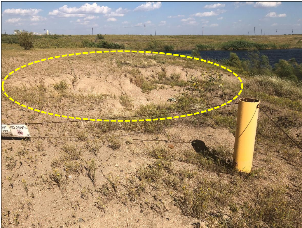
Photo 1. View looking east across erosion feature (circled) observed at northwestern edge of pond, near CPW-designated parking area.
