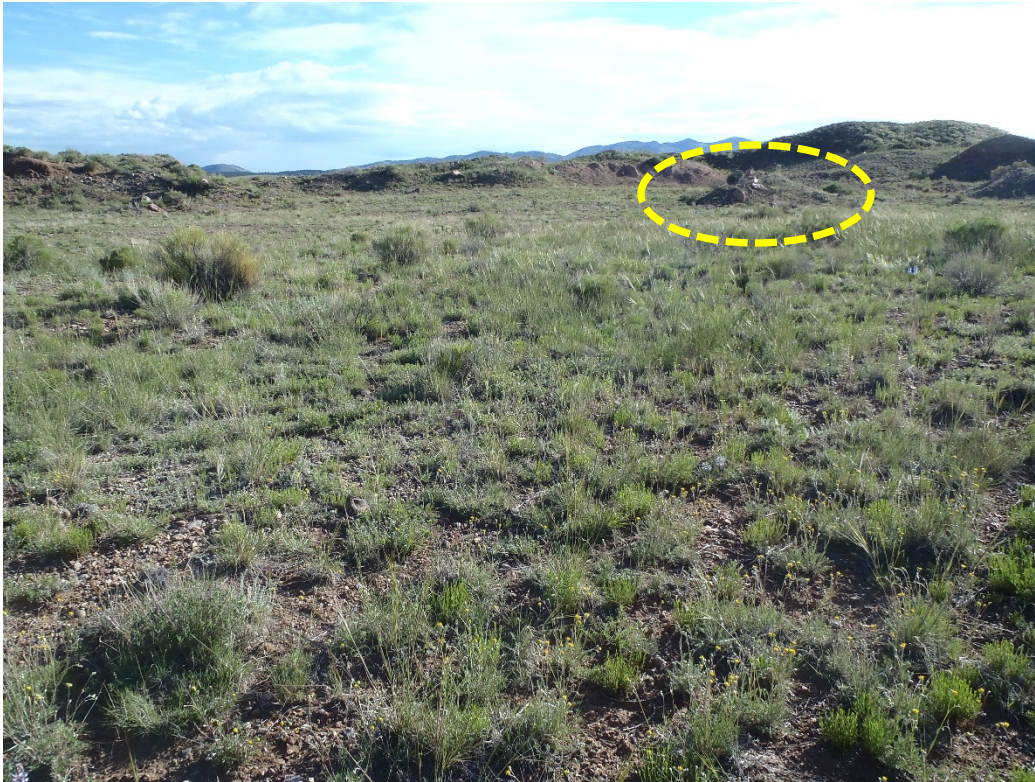
Photo 2. Pit floor, highwall on left, oversize rock stockpile circled (looking NE).
