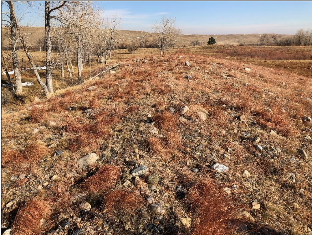
Photo 20. View looking east across reclaimed south mining area. Note all slopes graded 3H:1V or flatter and established vegetation consisting of grasses and some trees.
