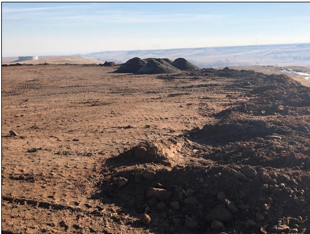
Photo 4. View looking east across top of backfilled portion of pit (upper lift) in north mining area. Note small stockpiles of imported material stored on top of lift.
