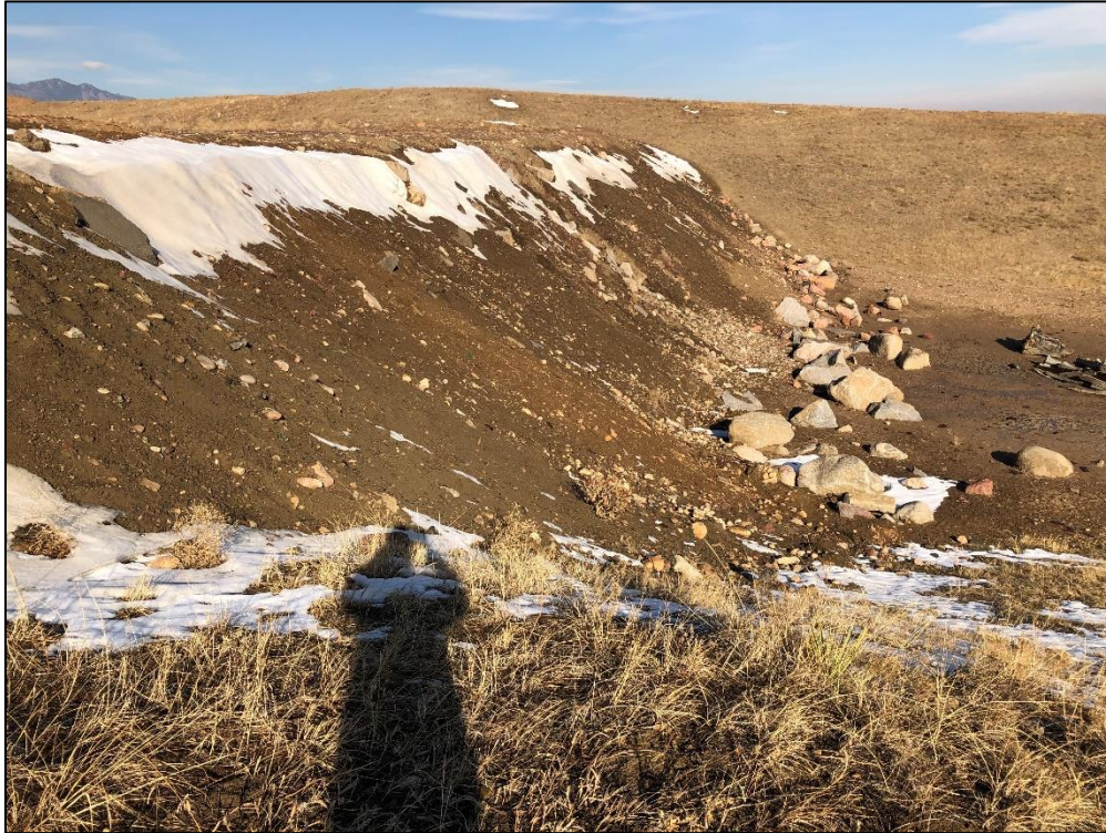
Photo 7. View looking north across eastern side slope of lower lift at approximate 1.5H:1V to 2H:1V gradient.
