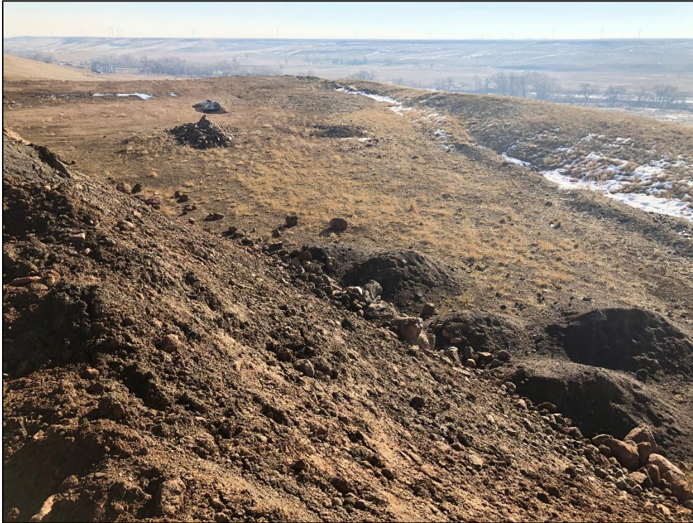
Photo 5. View looking east across top of lower lift of backfilled pit in north mining area. Note side slope of upper lift (in foreground) at an approximate 1.5H:1V gradient.
