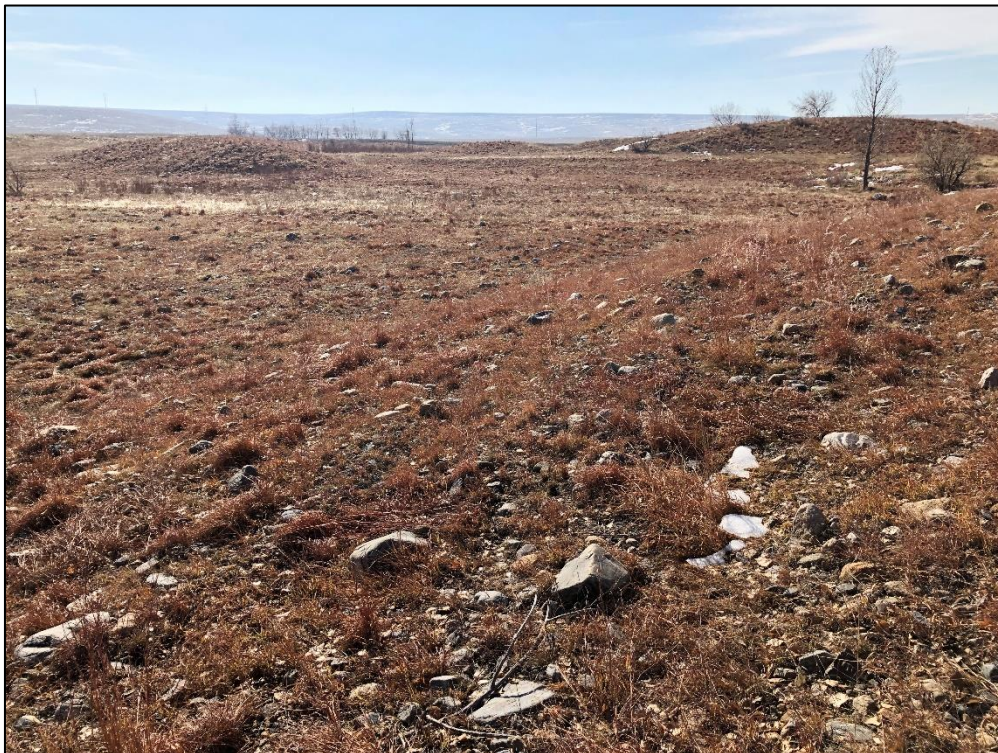
Photo 16. View looking southwest across reclaimed south mining area. Note all slopes graded 3H:1V or flatter and established vegetation consisting of grasses and some trees.
