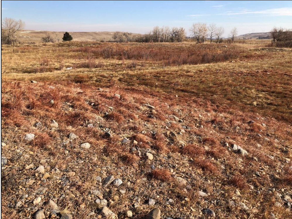
Photo 17. View looking southeast across reclaimed south mining area. Note all slopes graded 3H:1V or flatter and established vegetation consisting of grasses and some trees.
