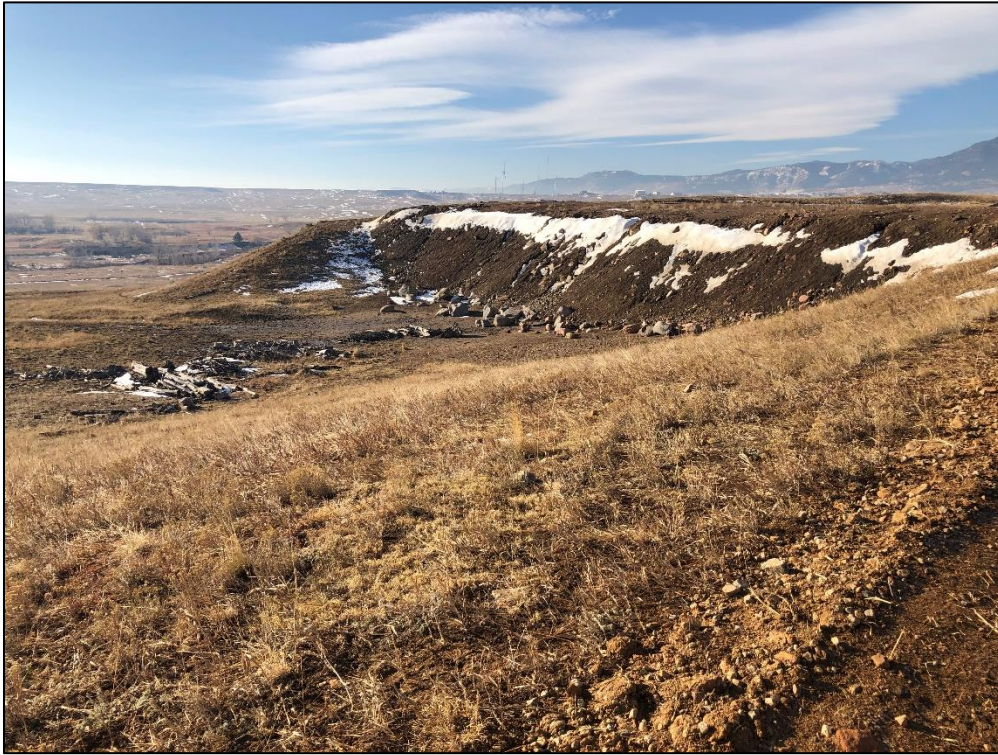
Photo 1. View looking southwest from access road across eastern portion of pit located in north mining area, which the operator is backfilling. Note eastern side of lower lift shown at right.
