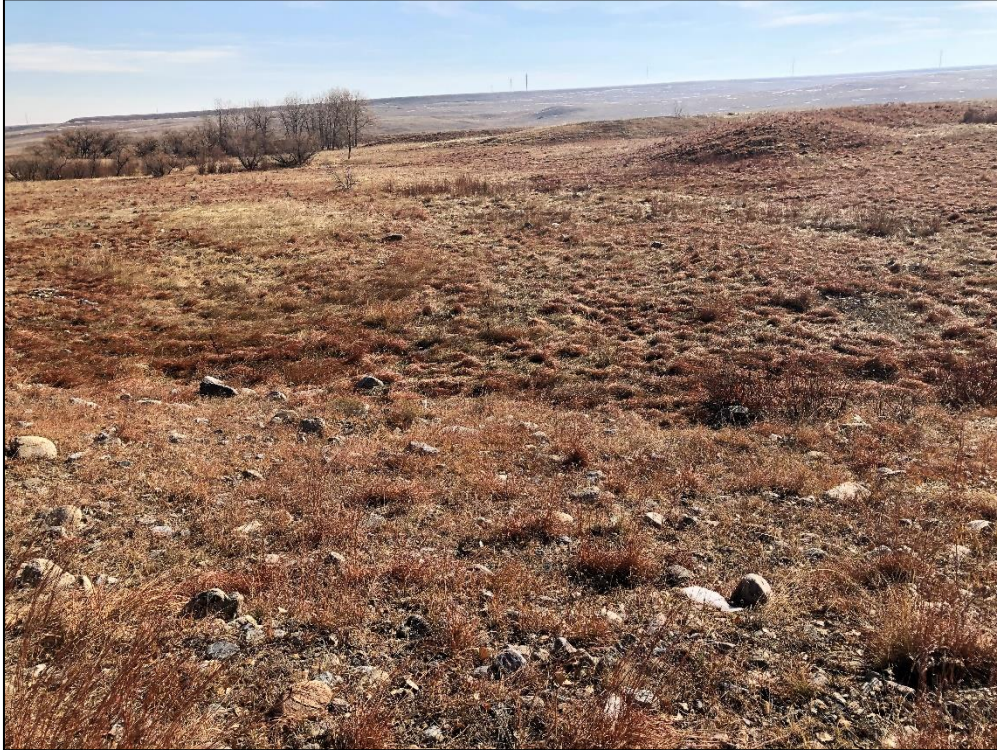
Photo 19. View looking south across reclaimed south mining area. Note all slopes graded 3H:1V or flatter and established vegetation consisting of grasses and some trees.
