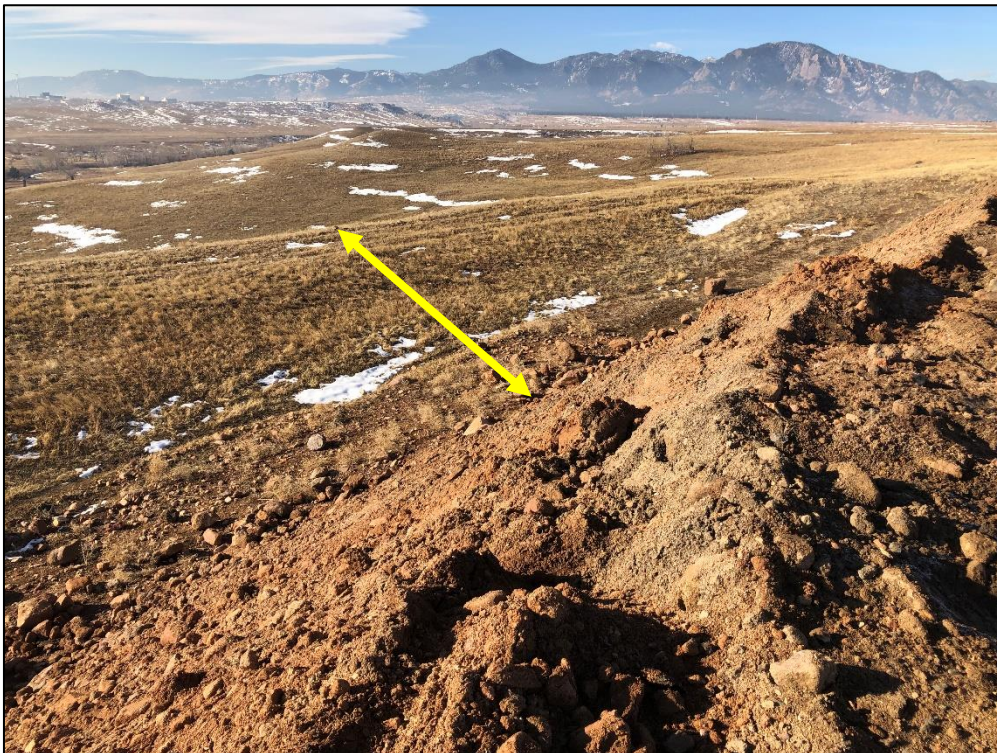
Photo 6. View looking west from top of upper lift of backfilled pit in north mining area, showing southern section of pit (indicated) which operator intends to continue backfilling, although not required by the approved reclamation plan.
