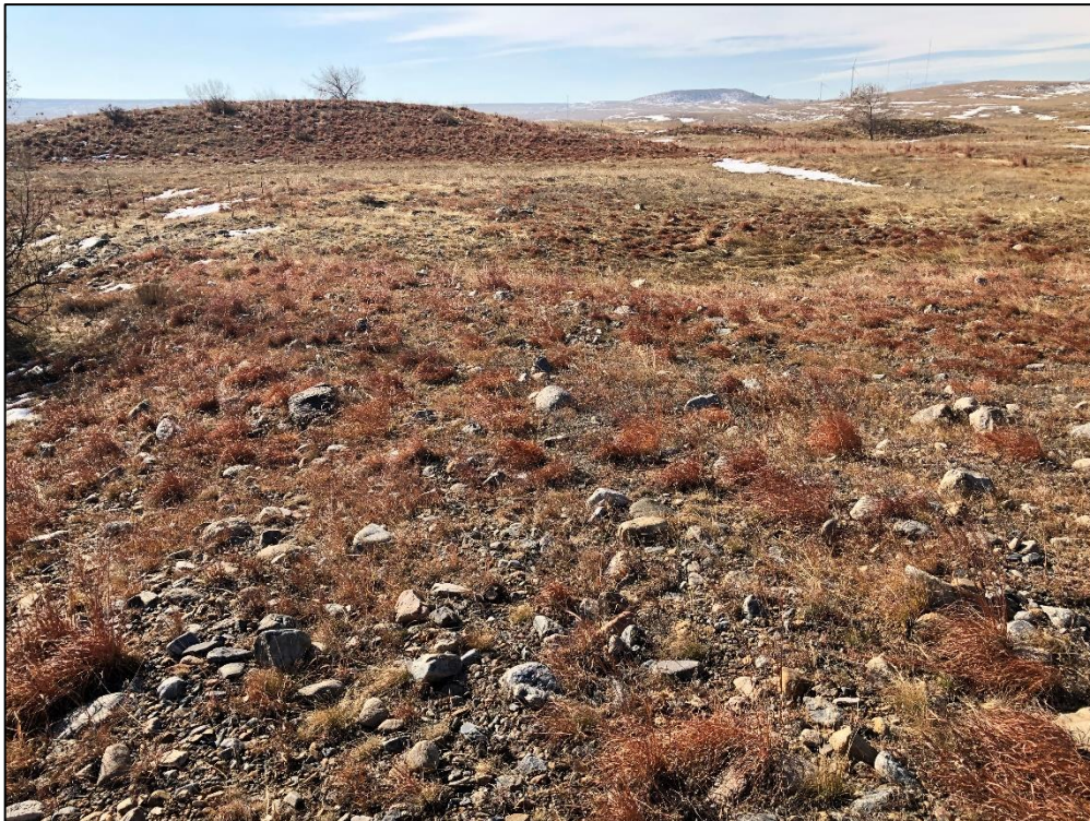
Photo 18. View looking west across reclaimed south mining area. Note all slopes graded 3H:1V or flatter and established vegetation consisting of grasses and some trees.
