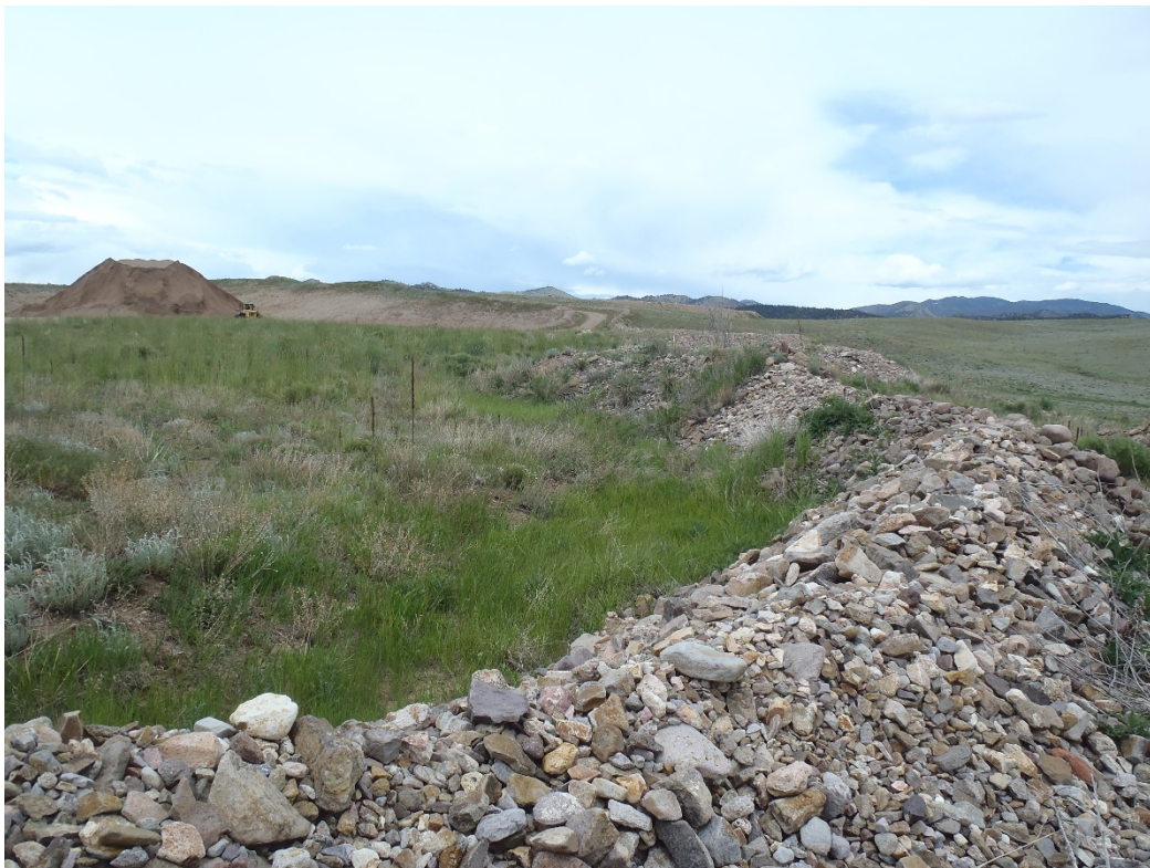
Photo 5. Rock check dam on the southwest corner of the site (looking east).
