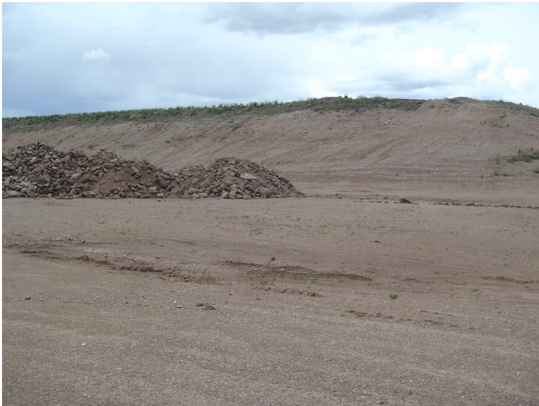
Photo 1. Highwalls (~25 feet high) appearing stable sloped at roughly 2H:1V (looking NE from pit floor).
