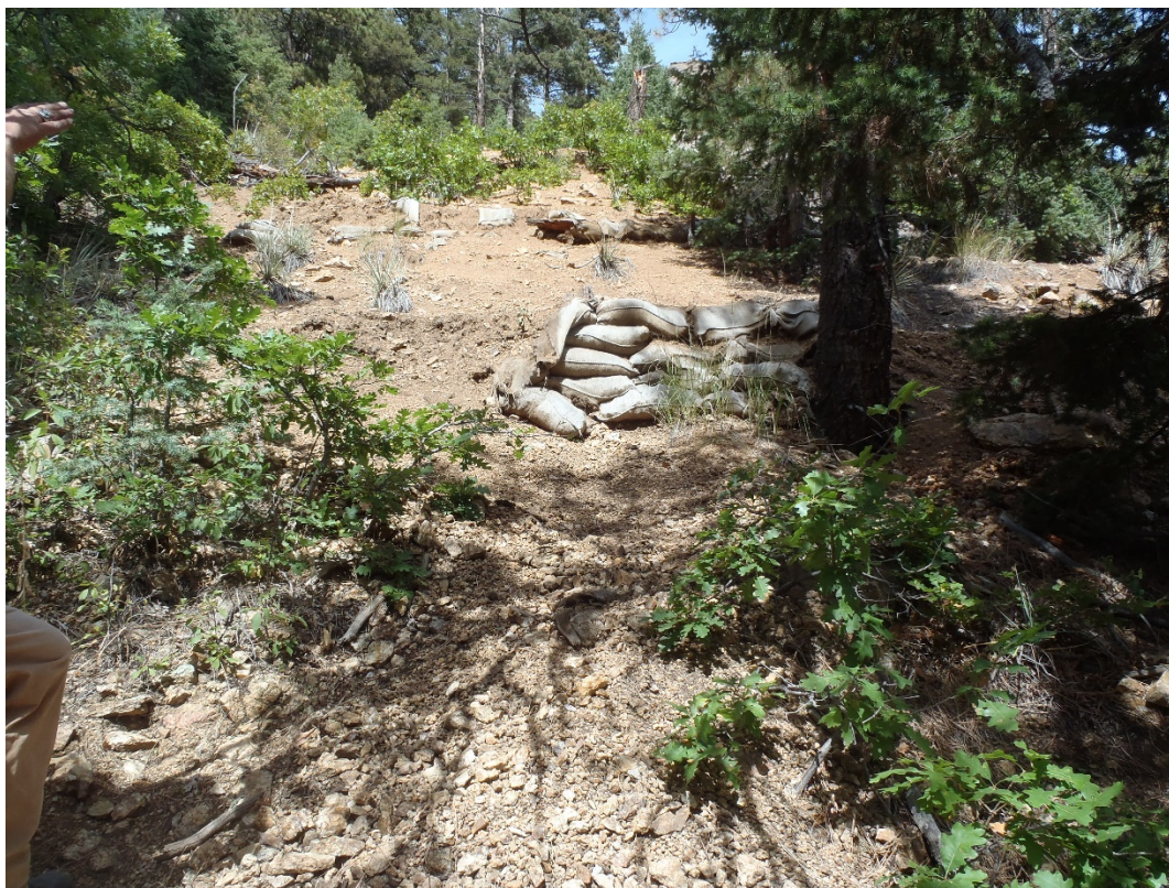
Photo 1. Stabilization of cast-off material (looking west from downhill & east of Discovery Pit #2).
