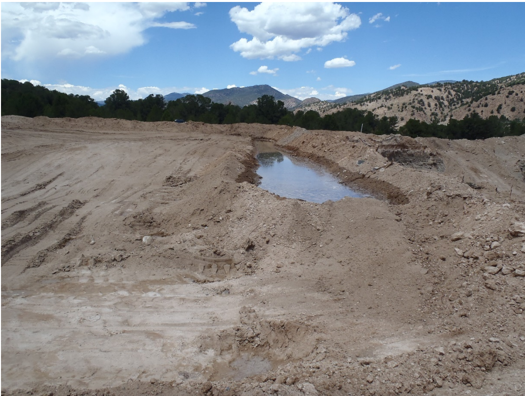
Photo 1. Standing water observed in trench near the crest of the highwall (looking NW).
