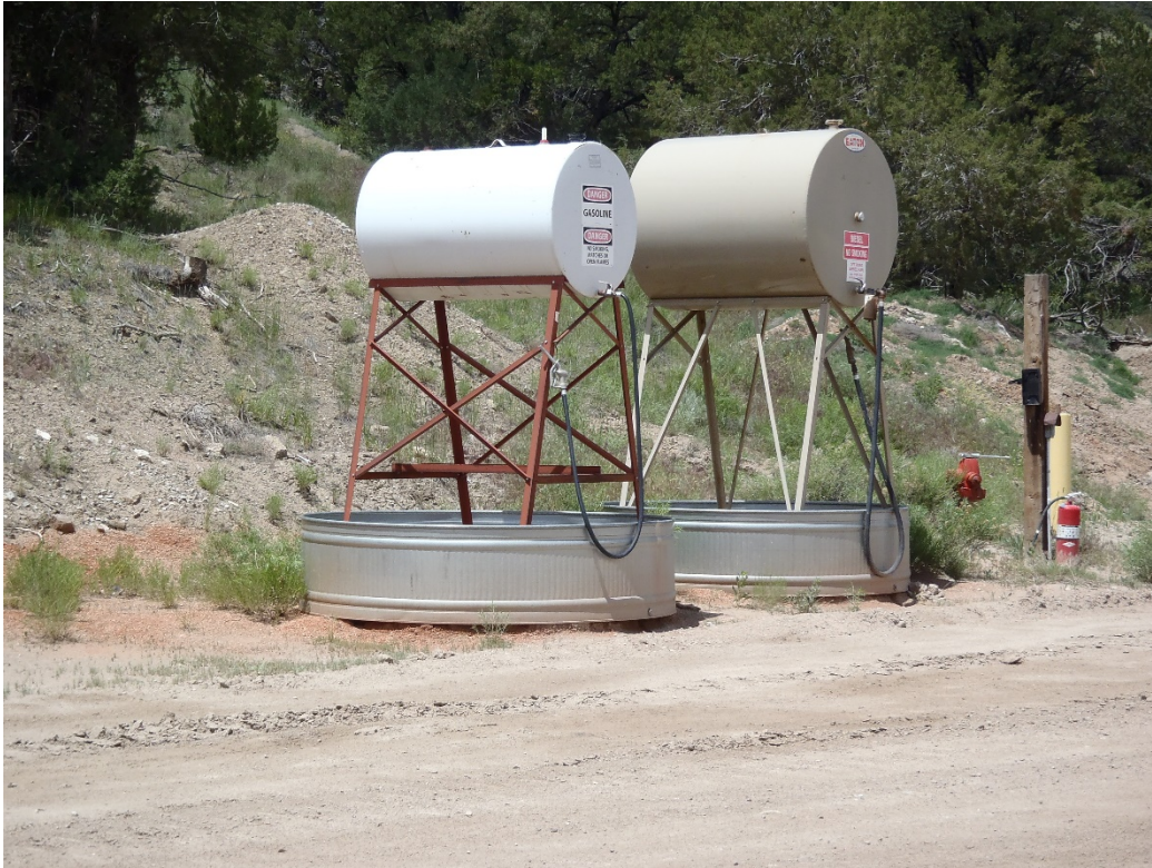
Photo 8. Fuel storage secondary containment.
