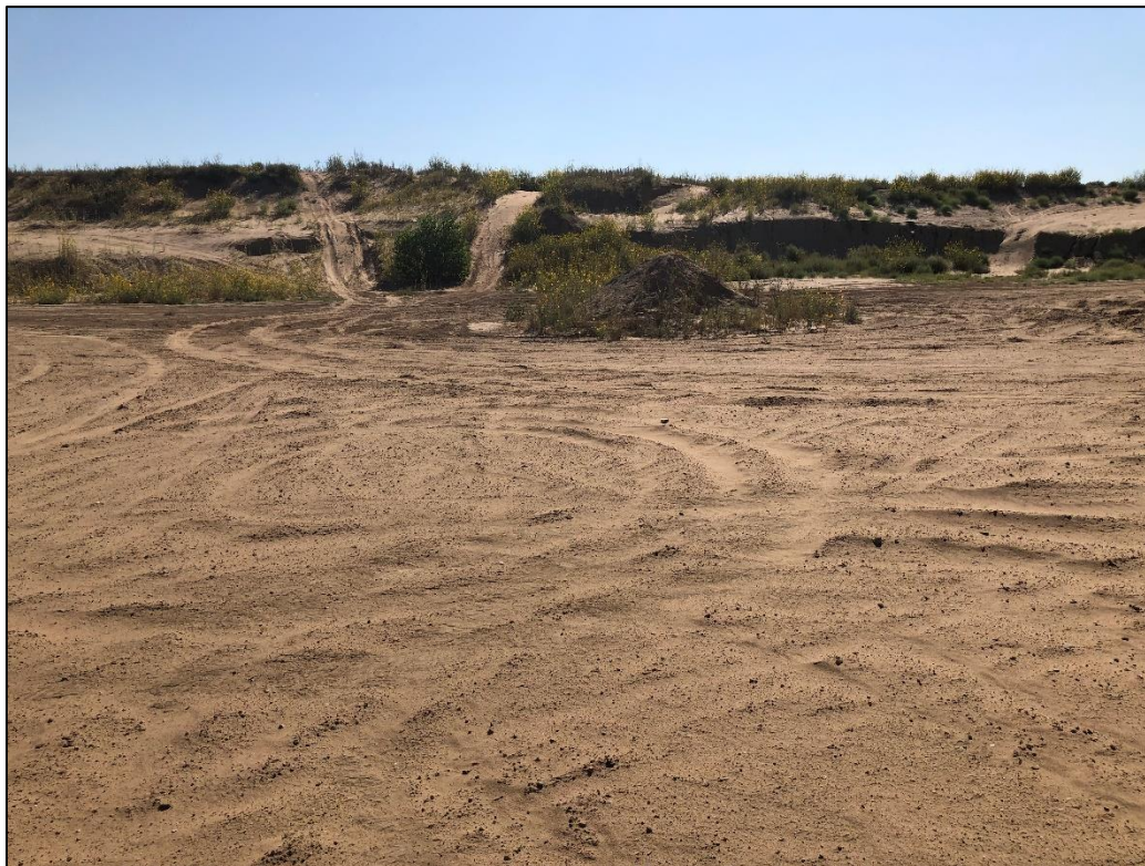
Photo 3. View looking east across pit area, showing small material stockpile stored on pit floor and eastern pit wall (in background) with dirt bike trails across its slope.
