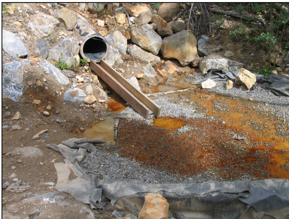
Figure 2. View of current mitigation at lower sump using crushed limestone in an EPDM lined sump with concrete headwalls and 0.5-foot H-flume (out of view to the right). Note 24-inch HDPE discharge pipe and wooden directional flume for Deadman Gulch bypass flow. Photo by Wayne Pandorf (DOWL) on August 5, 2016.
