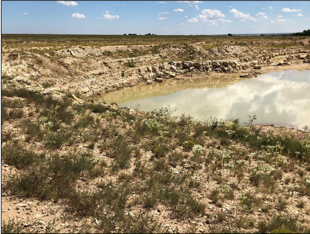
Photo 15. View looking southeast across pit from top of northern pit wall. Note ponded water present on pit floor. Also note pit wall approximately 12-15 feet in height with near vertical to 1.5H:1V slopes in this portion of the pit.
