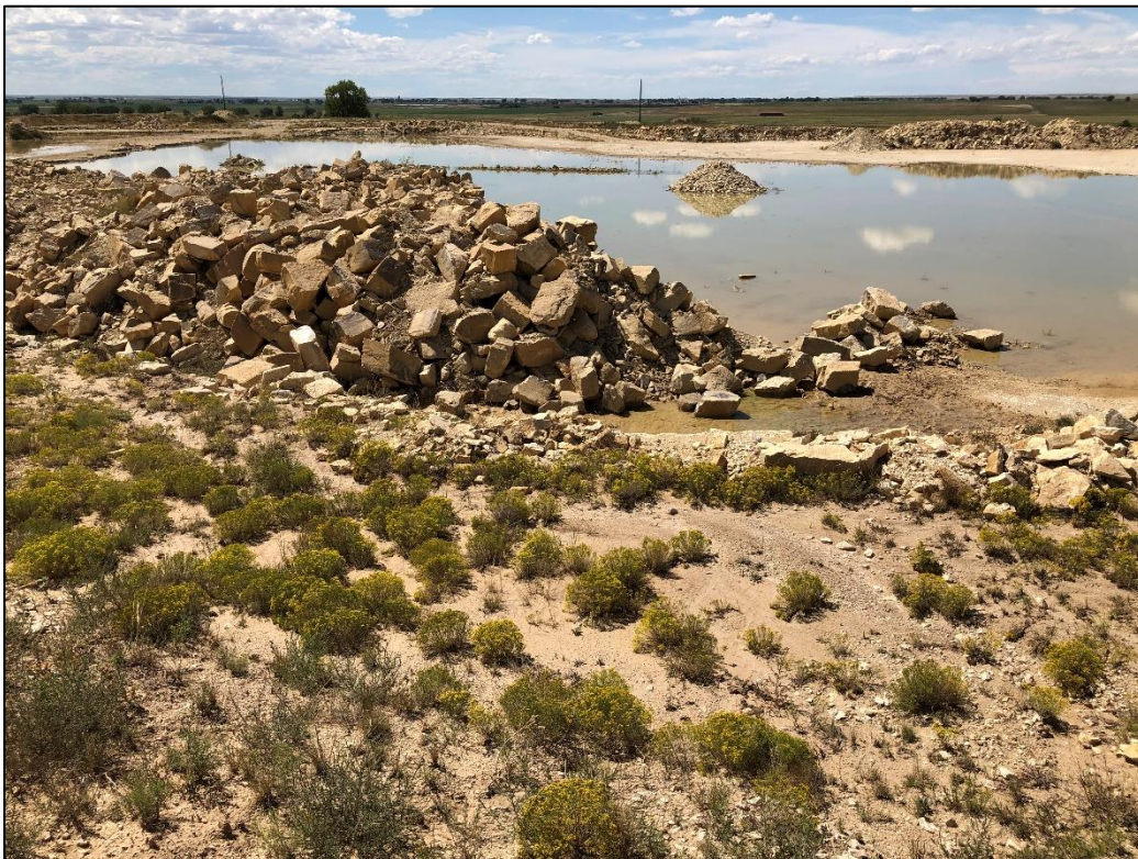
Photo 18. View looking southwest across pit from top of eastern pit wall. Note ponded water present on pit floor. Also note material stockpiled on pit floor.
