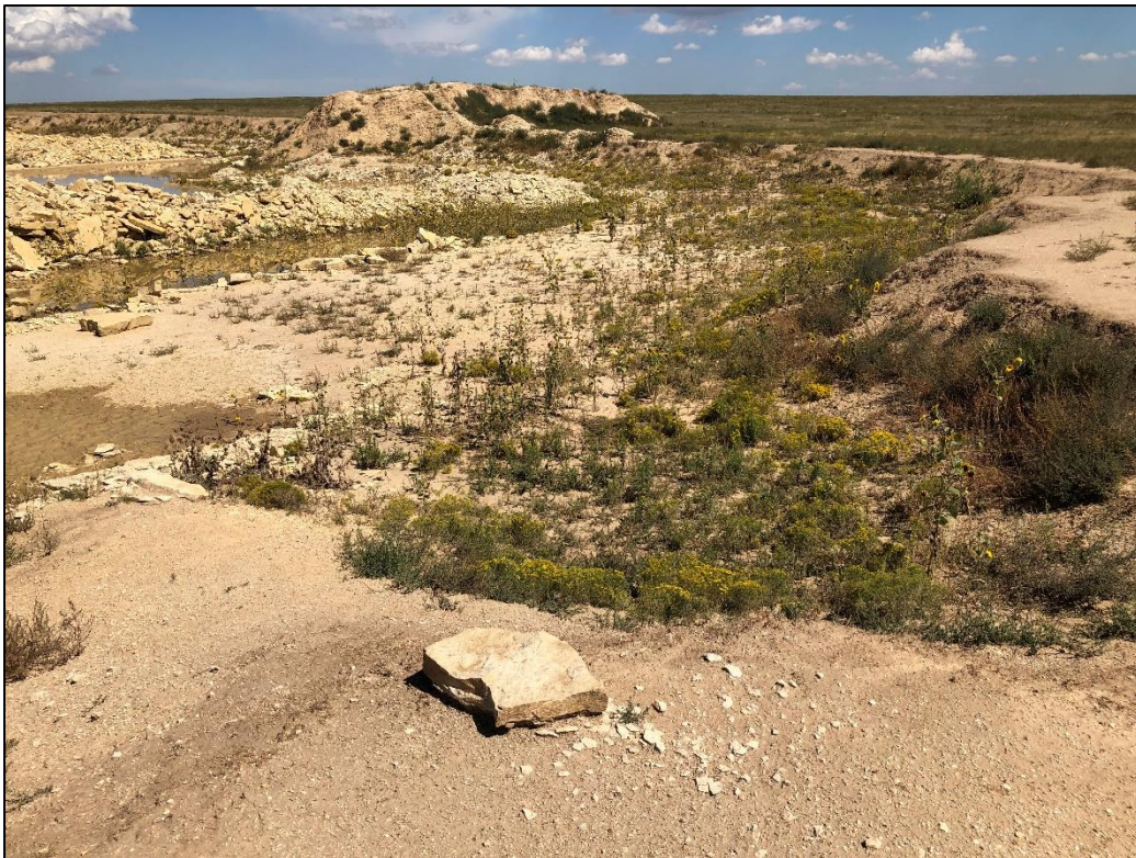
Photo 22. View looking east across southern pit wall. Note pit wall approximately 4 feet in height with approximate 1H:1V slopes in this portion of the pit.
