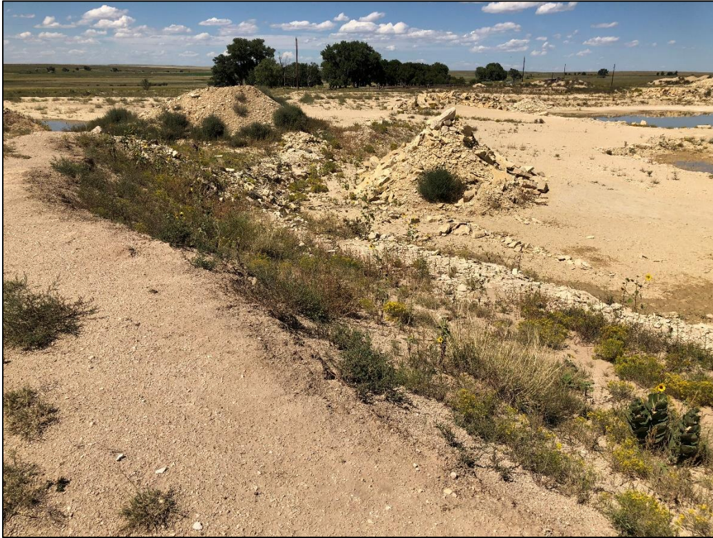
Photo 23. View looking west across southern pit wall. Note pit wall approximately 4 feet in height with approximate 1H:1V slopes in this portion of the pit. Also note material stockpiled at southwestern edge of pit.
