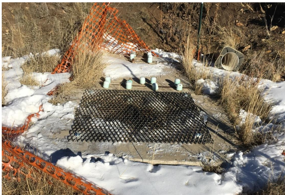
Photo 10. Open Borehole 2 after safeguard installed, looking north. Photo taken 11/19/18.
