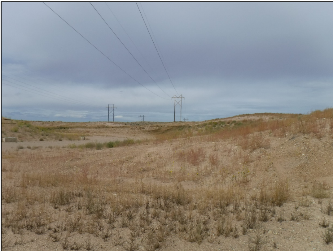
Photo 6: Graded high wall slopes to 3H:1V or less
