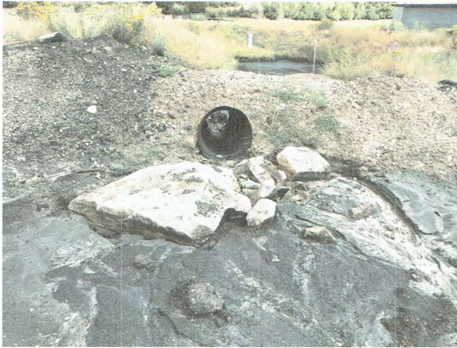
Pic. 3 – Riprap at pipe entrance to east pond.
