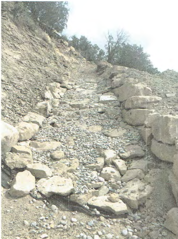
Pic. 2 – New riprap section of Reach 1 channel.
