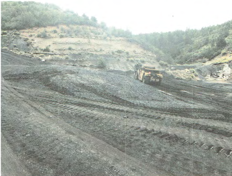
Pic. 4 – Waste material at base of embankment/waste pile collected via excavator.
