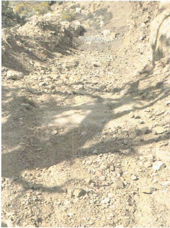
Pic. 3 – Upper section Reach 1 channel awaiting shot-crete lining.
