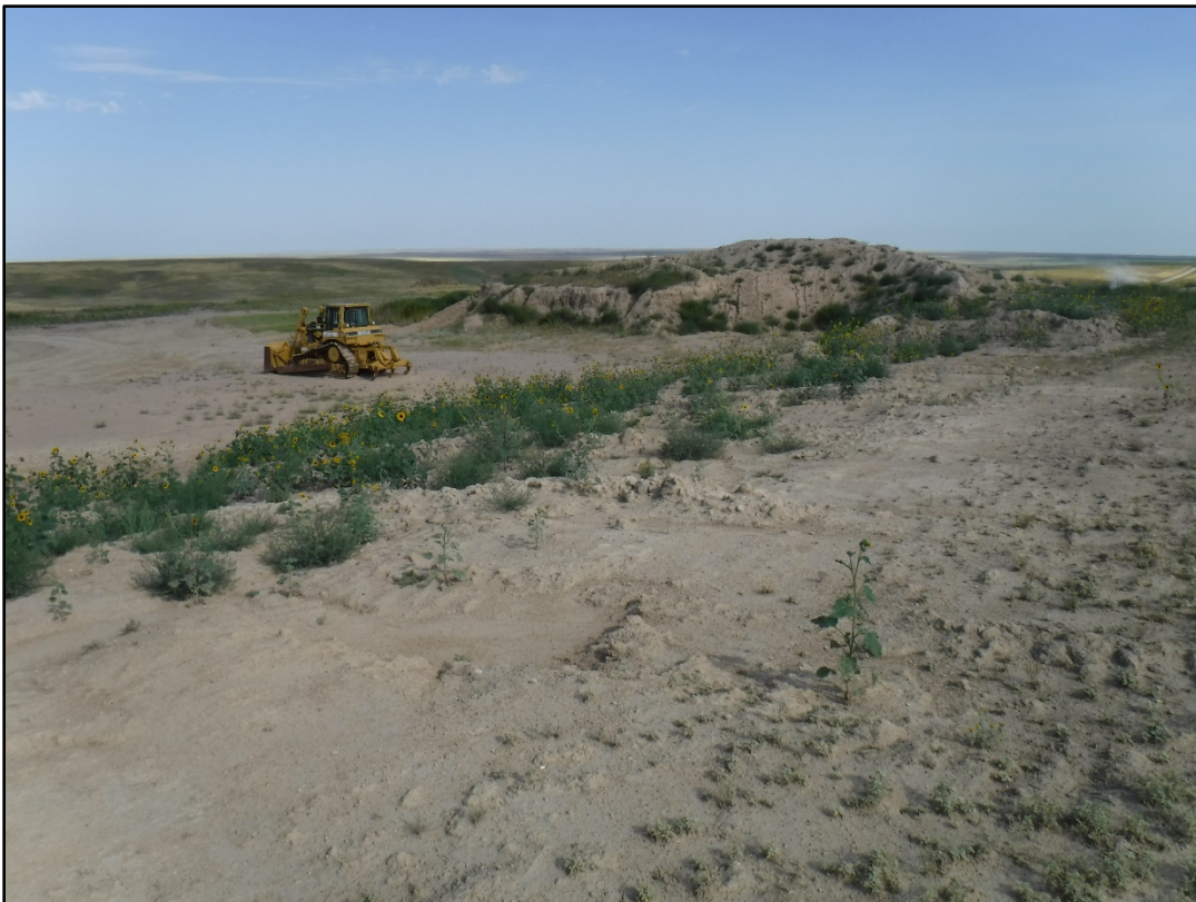
Photo 6: Highwall, center of picture, showing rilling occurring that is contained on pit floor
