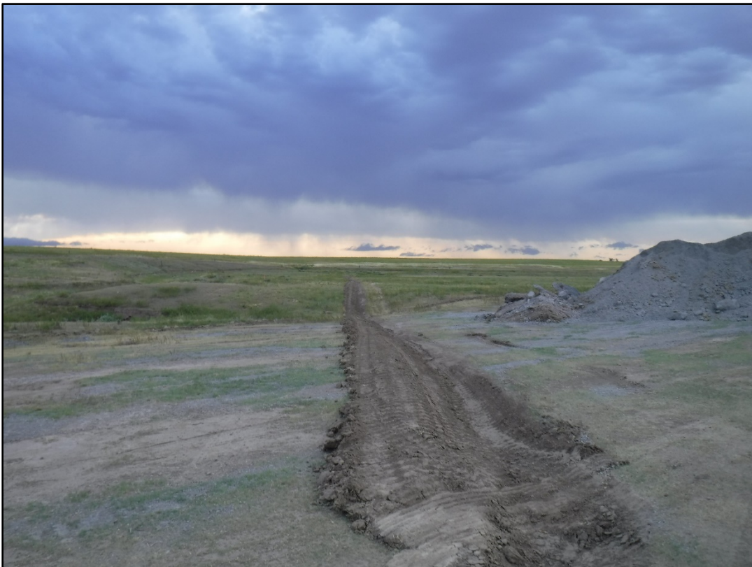
Photo 4: Typical section of the run-on/-off control berm that follows permit boundary
