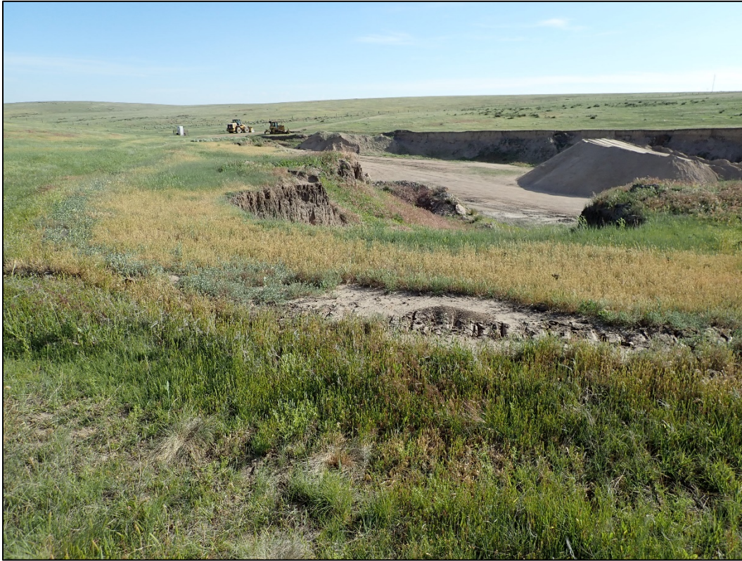
Photo 5. Head cut erosional feature along west/southwest side of the pit; looking northeast.
