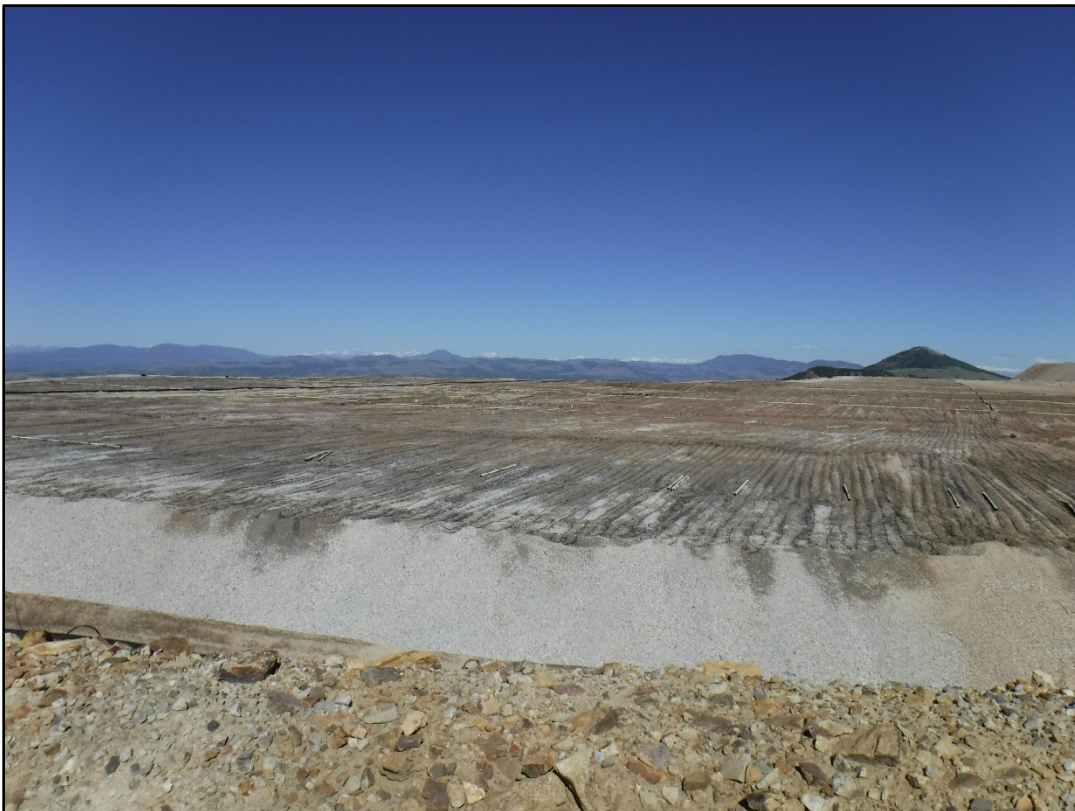
Photo 8: SGVLF active leaching areas appeared to be well-ripped to minimize ponding, 9900' level
