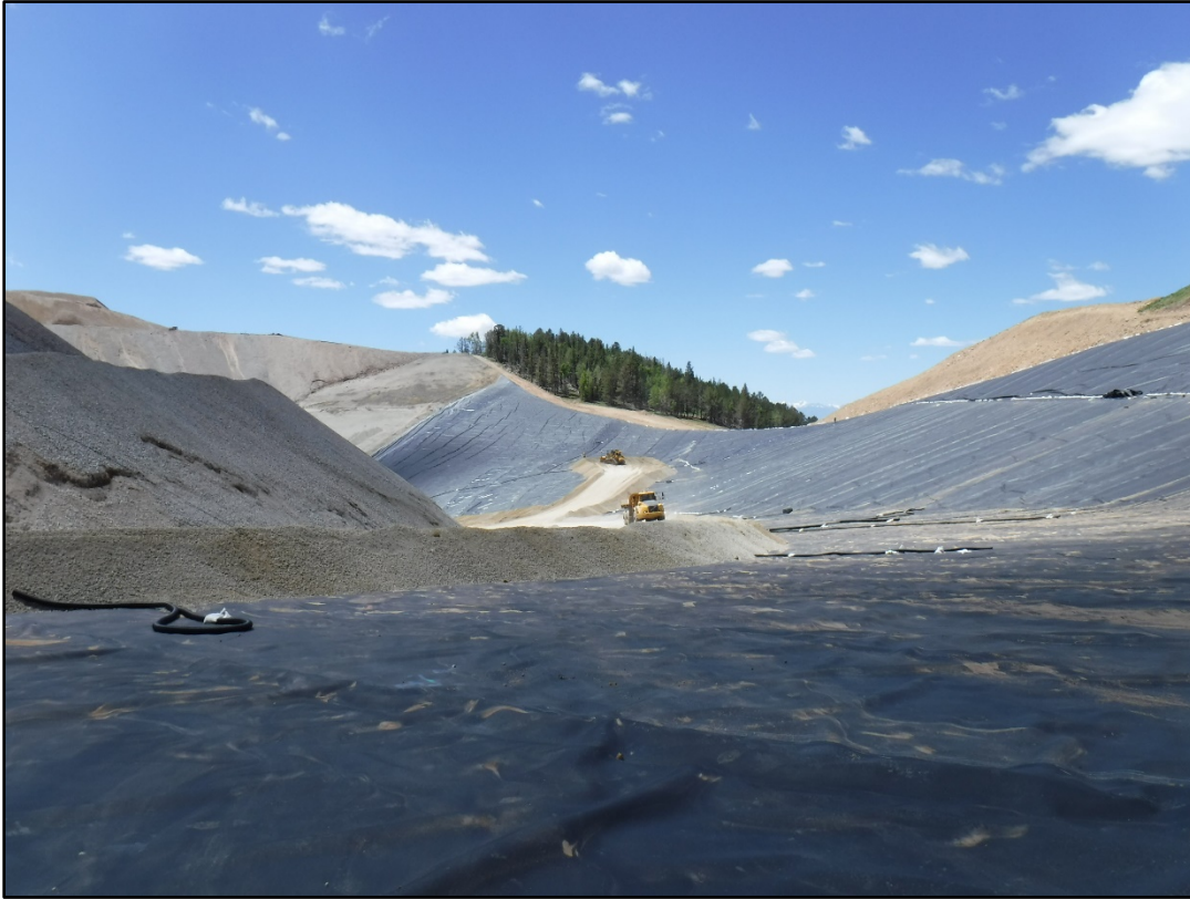
Photo 19: VLF 2 Phase 2 construction, DCF hauling and placement
