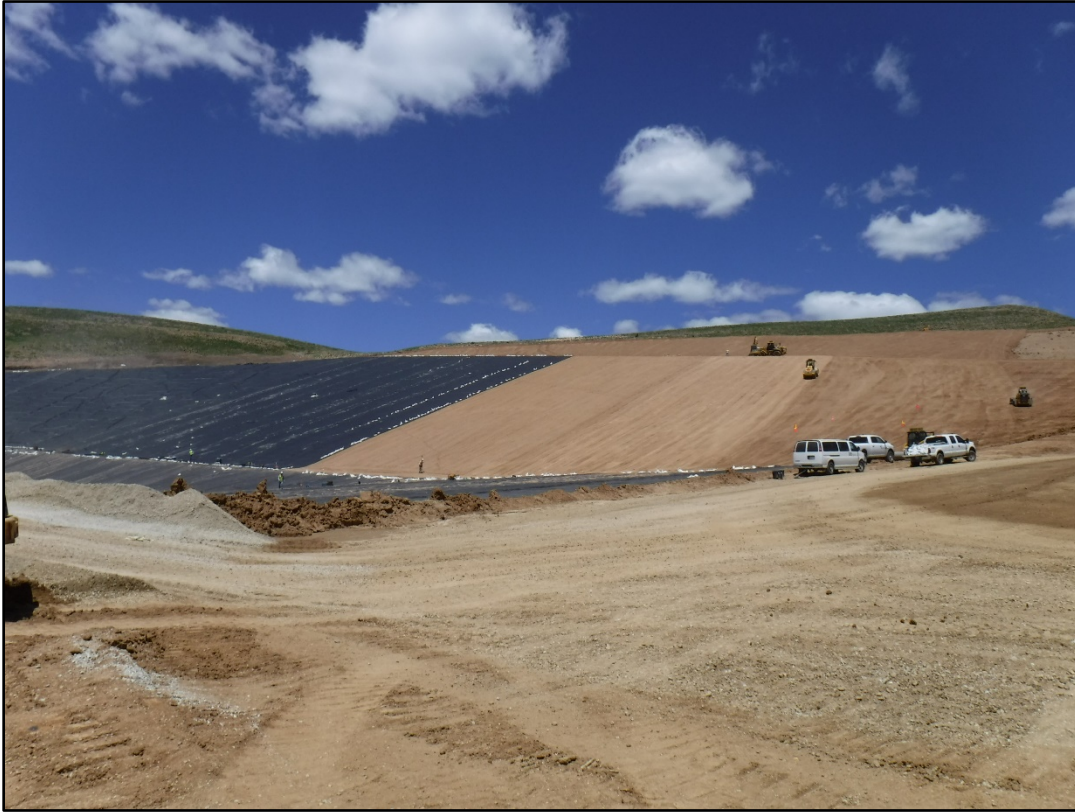
Photo 17: VLF 2 Phase 2 construction, panels deployed in morning and subgrade prep for additional liner placement
