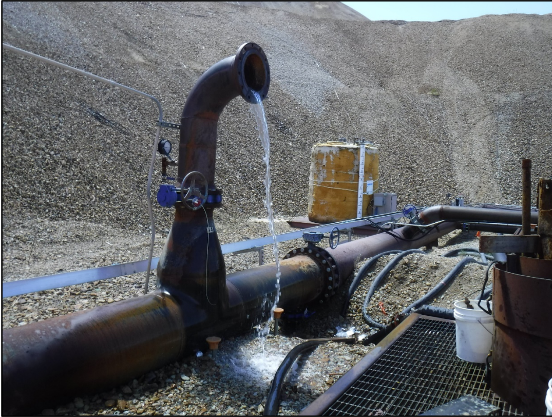
Photo 15: Solution bypassing the gate valve at the 303 pump Phase I, AQVLF
