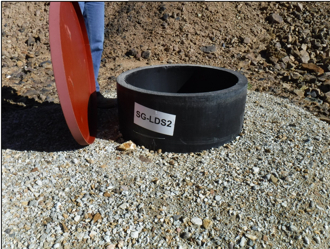
Photo 1: Leak Detection System Sump, SG-LDS2 (dry)
