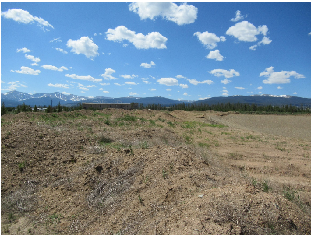
View of topsoil stockpiles stripped ahead of the highwall looking south
