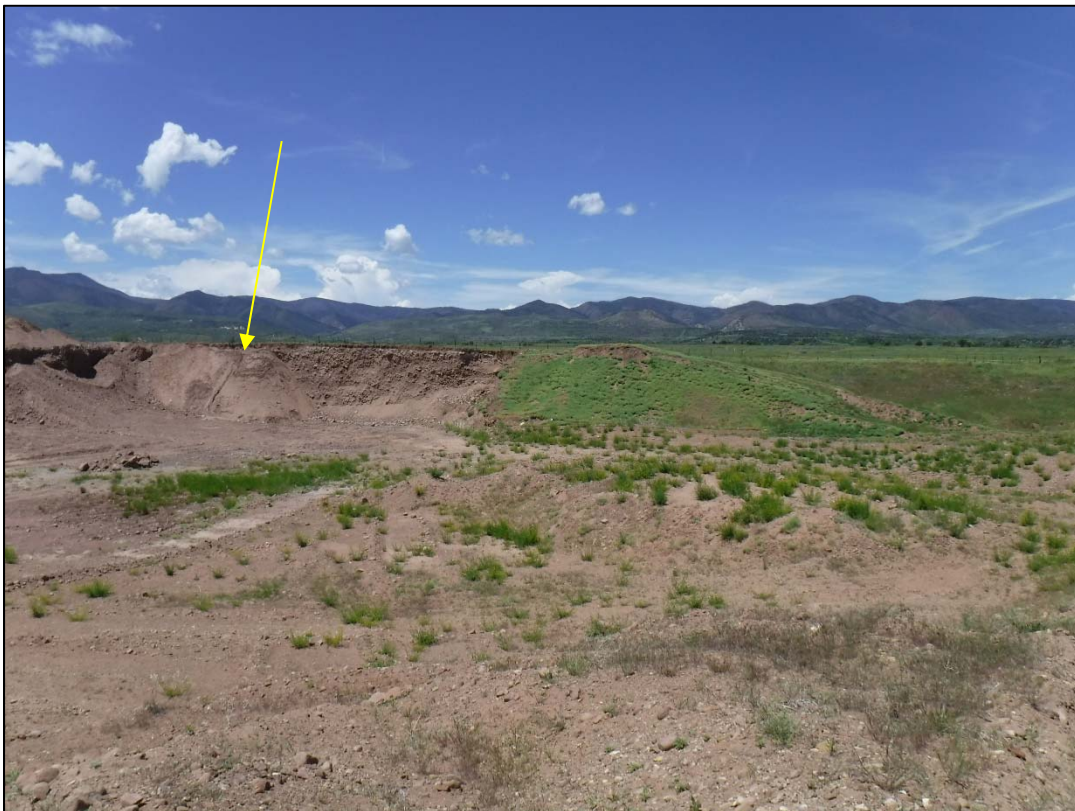
Photo 4: Looking at the west pit wall, arrow marks material being placed to reclaim highwall, topsoil pile center of picture with vegetative cover
