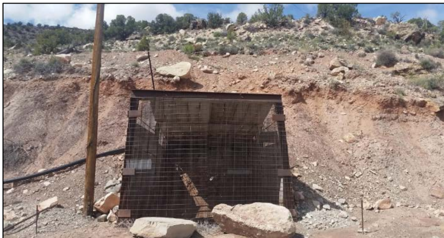
Figure 9: The Sunday Mine Portal, view looking south. The portal has been backfilled with rock for approximately 20 feet, and is also gated. This portal will be opened up this summer, but it will only be used as a secondary escape way and ventilation draw point.
