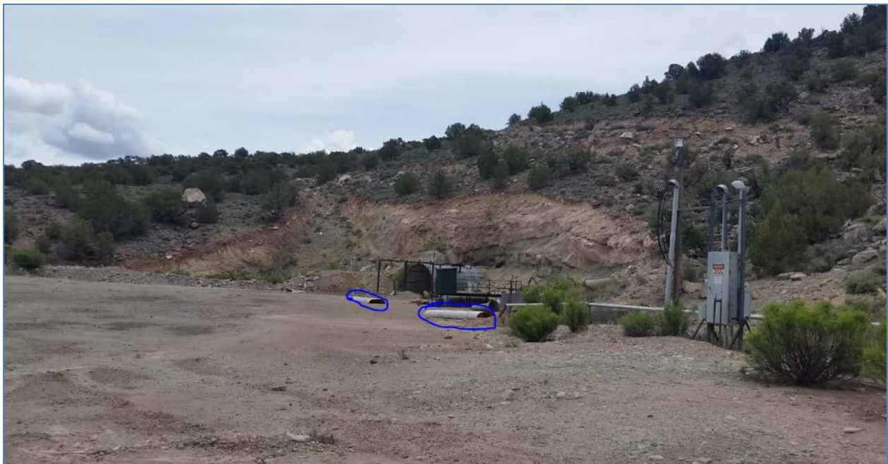
Figure 29: looking Southeast across the dump towards the portal of the Topaz mine. The site was generally tidy, with few if any weeds having emerged yet this year. The portal has been backfilled. There are some fiberglass ventilation ducts (blue circles) that have blown off of a stack. They should be disposed of if they aren't to be used soon.
