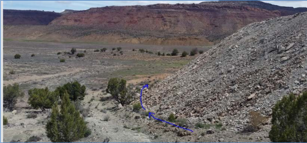
Figure 16: After inspecting the Carnation mine, we walked back along the toe of the Sunday dump. There was no sign of seeps at the toe of the dump. There was one place where there was substantial erosion that was caught by the secondary containment berm. I believe this erosion dated back to a documented storm event in 2014, caused by a breach in the berm at the top of the dump, which was subsequently fixed. I think the erosion has been arrested by repair of the berm, but will continue monitoring to see if it continues. The blue arrow shows the path we walked back to the entrance of the mines.
