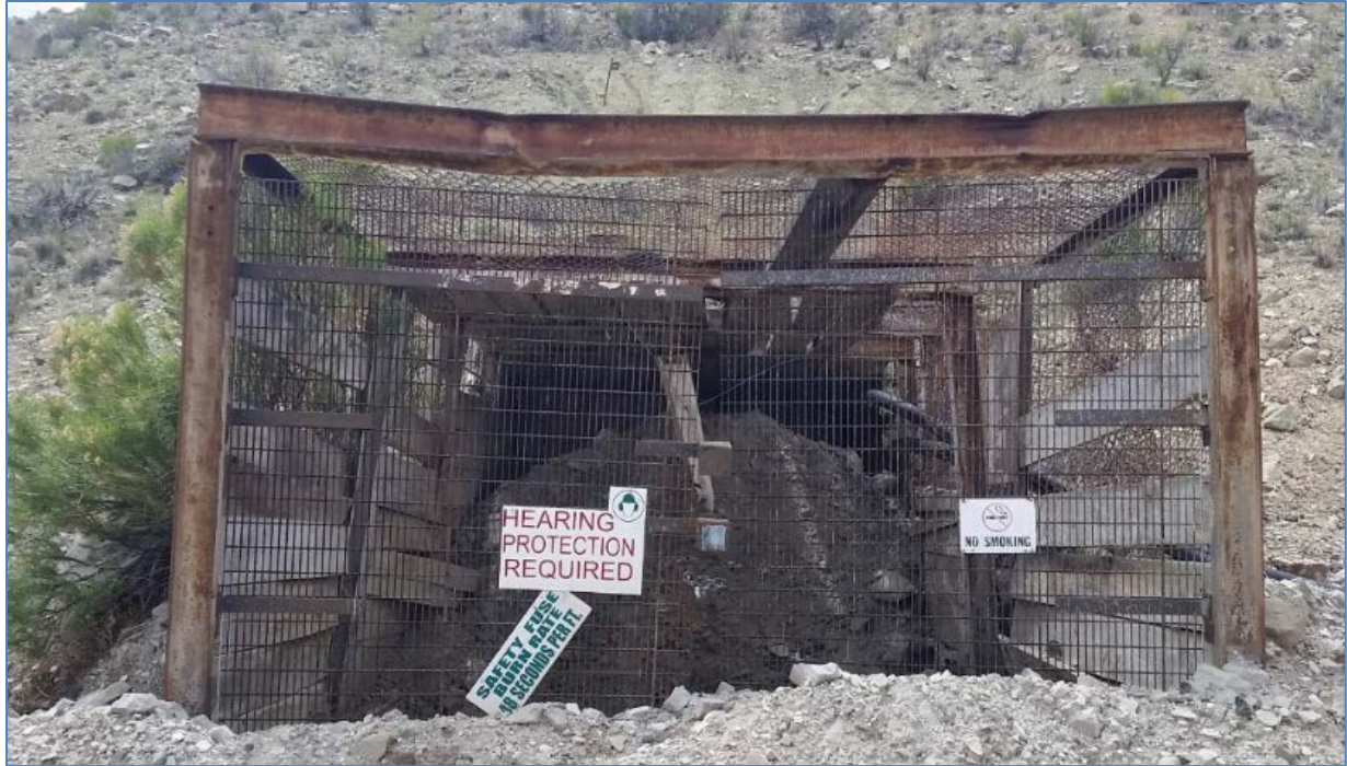
Figure 26: The portal of the West Sunday Mine. This portal has been backfilled about 20 feet back, in addition to the gate, top prevent trespassing. It is not slated to be opened up for the exploration project this year.
