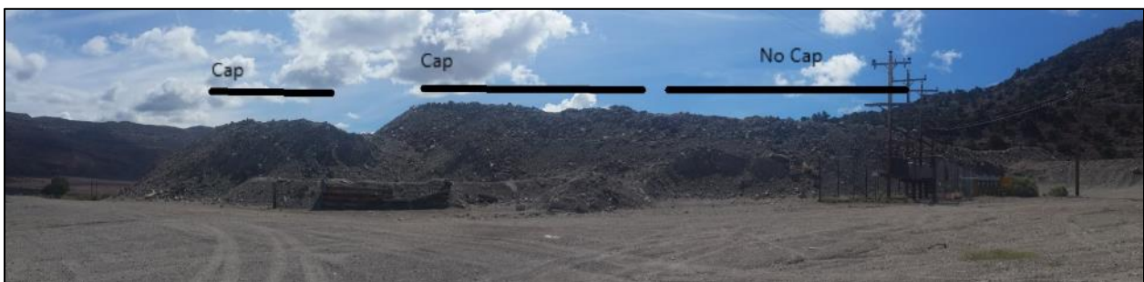
Figure 2: Panoramic photograph looking east from map 2 point 1 showing the low-grade stockpile on the east end of the Sunday's surface facilities that will be capped with barren waste rock. Also visible is de-energized transformer substation for the Sunday. There are no plans to re-energize the substation.
