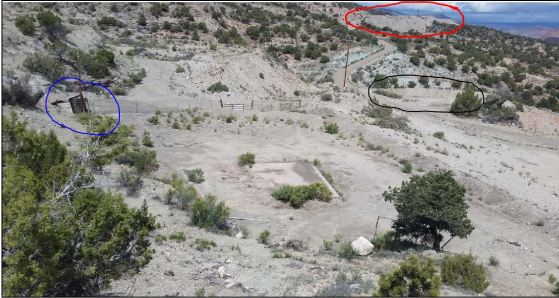
Figure 14: A view of the Carnation Mine (portal in blue circle). The only use for this is an alternate escapeway. Everything beside the portal should be reclaimed, as should the portal if they decide that they no longer need it. The pad in the foreground was probably for scales or a hopper. The black circle is a storm water pond that I have seen brim full or breached before, but today it is bone dry inside, despite it having appeared to have rained only a few days prior. The red circle is the St. Jude Mine. The county road that goes over Gyp Ridge is in the mid-ground.
