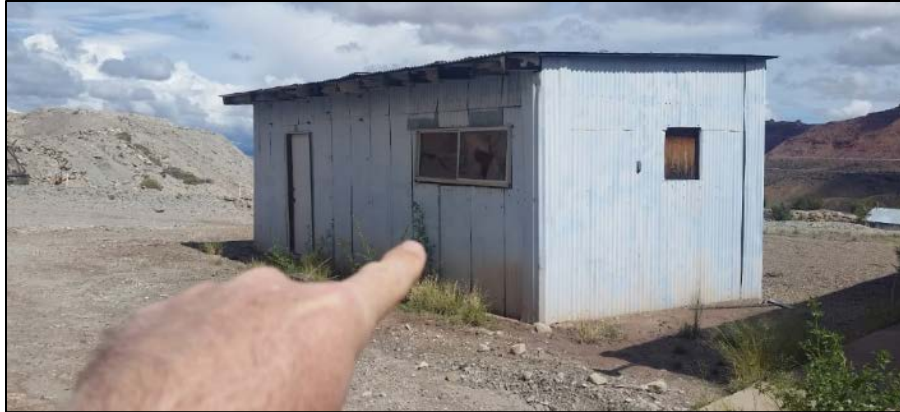
Figure 8: Broken windows and door in one of the outbuildings at the Sunday mine. I believe that this building was a scale house at one time. Will check to see if a sprung door is acceptable for an empty building in lieu of a lock, alternately consider tearing building down if not needed.
