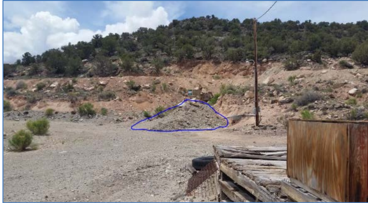
Figure 23: Looking southeast at the portal of the St. Jude Mine. Waste rock has been pushed into the portal and piled up outside of it to prevent unauthorized access inside after some theft and vandalism back in 2011. This material will be removed when the portal is opened this summer. This portal will be the main access point to the underground workings of the Sunday Mines Complex for the underground sampling and characterization activities. It will also function as a draw point for ventilation air.
