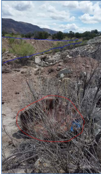
Figure 18. A view looking east along the toe of the Sunday Dump. The blue lines show the secondary containment berm at the toe. The black line circles material that eroded off the top of the dump and deposited at the bottom (see last photo). The black line shows a crushed 55 gallon drum. The drum will need to be picked up and disposed of. There was no sign of oil staining next to the drum, or indication that it contained any product.
