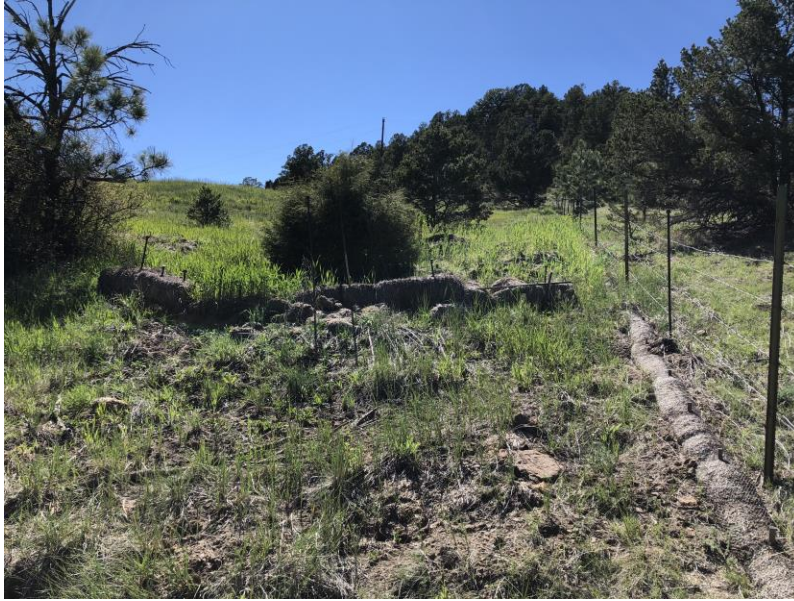
Sediment BMPs at former Golden Eagle site
