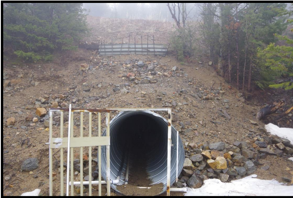
Photo 5: Portal entrance into the Times Mine; County Road 52 above
