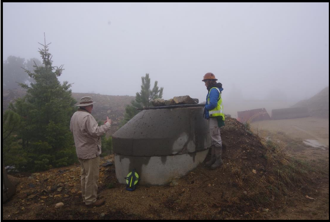
Photo 3: Concrete manhole around the Wynona mine shaft (collapsed and backfilled)
