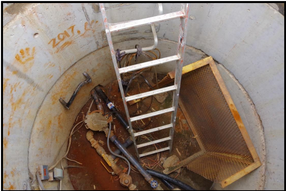
Photo 4: Inside Wynona Mine Shaft manhole; Well casing into shaft at upper left
