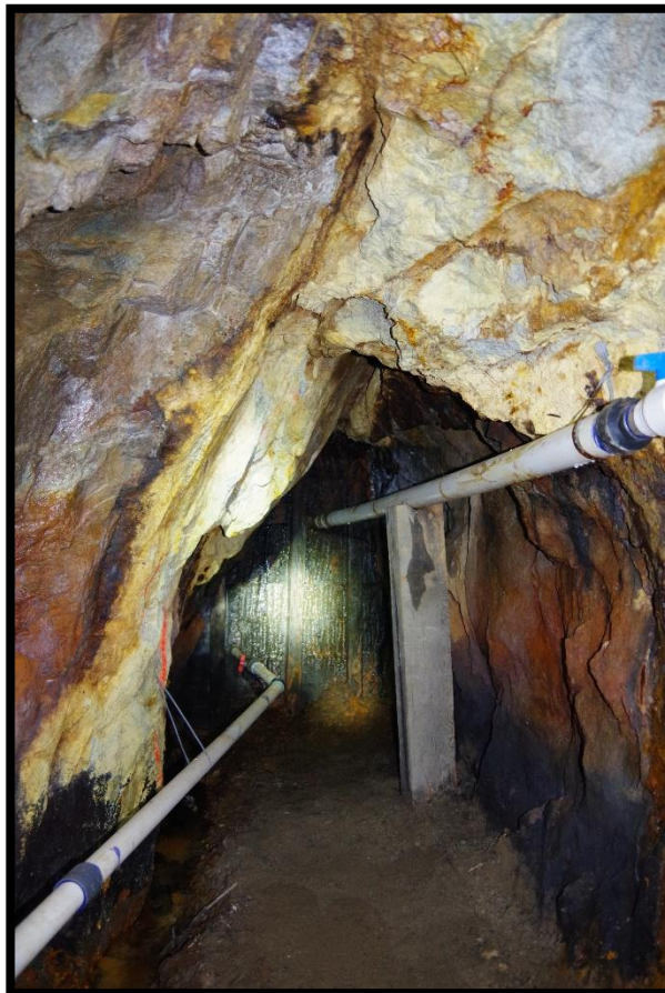
Photo 8: Piping in drift and into bulkhead; Note off-white alteration zone
