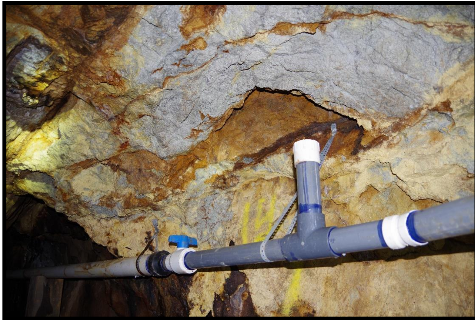
Photo 7: Upper pipe in Times Mine drift along vein; Note closed valve and Tee
