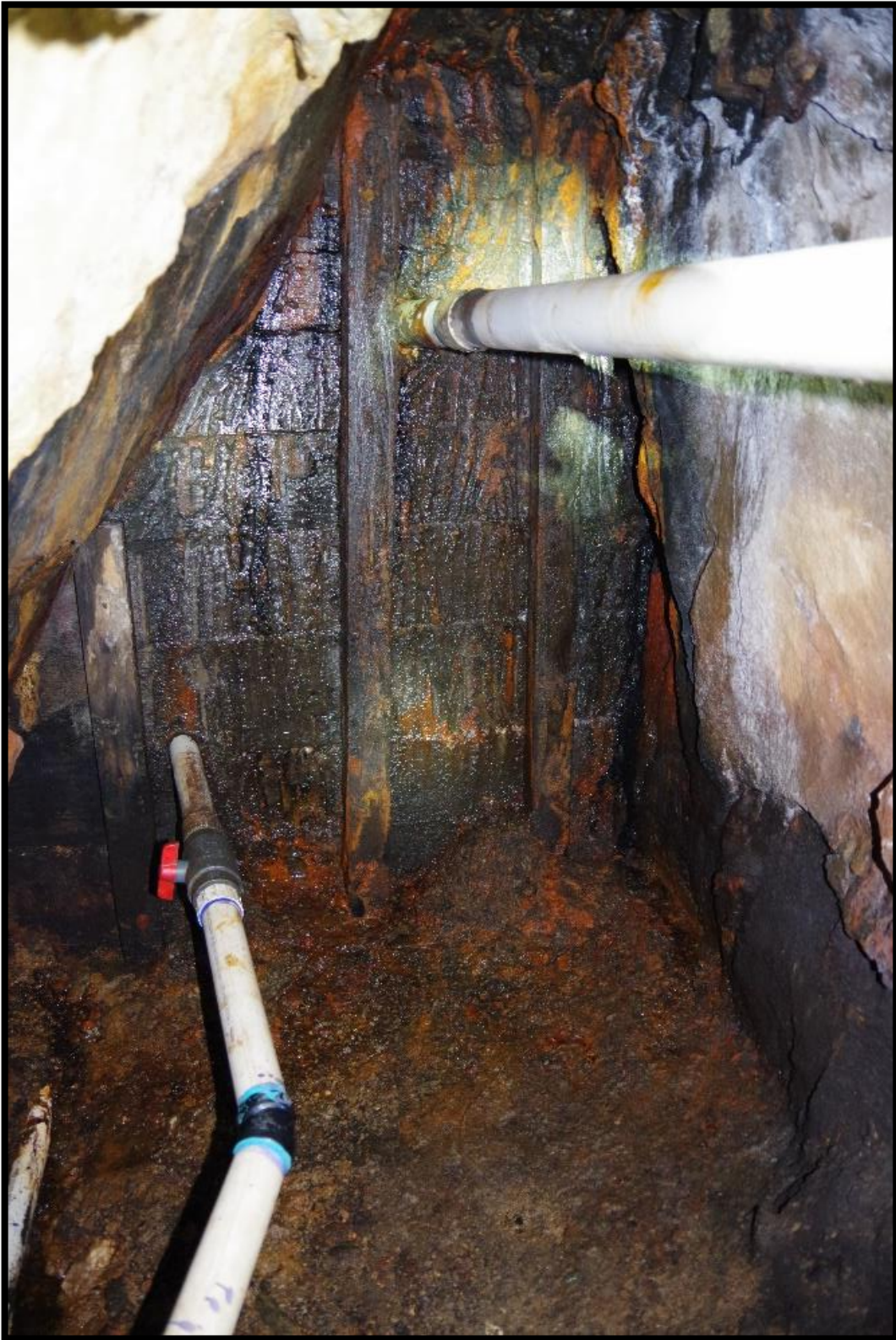
Photo 9: Bulkhead overview; Note wood forms remain in place and altered rock removed
